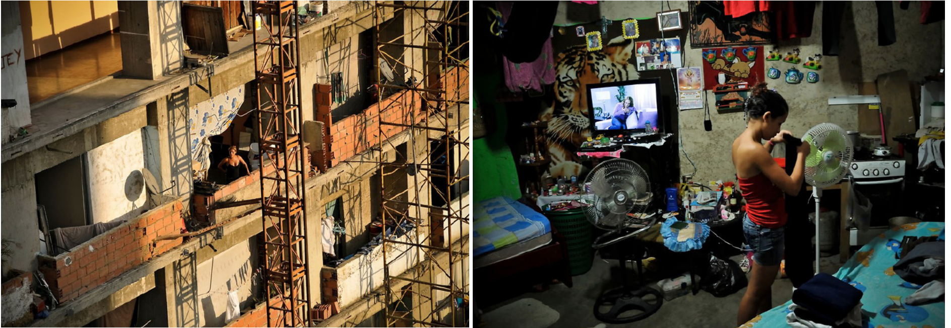
Images 4.18-4.19 Despite the arduous task of hauling building materials up several stories, and the concerns for safety, citizens have pressed on, slowly taking over floor after floor of El Torre de David, constructing walls and taking up residence. Images by Meredith Kohut for the New York Times (nytimes.com)
