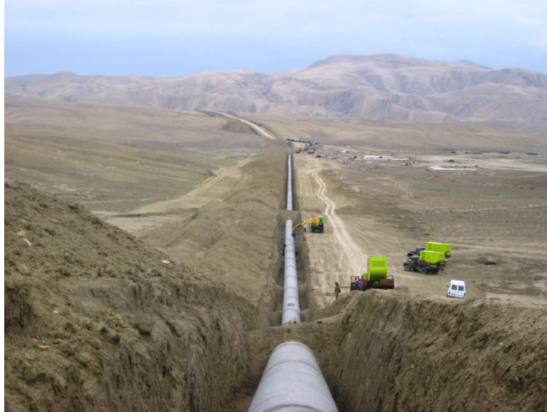
Figure 4.2 Construction of the Oğuz-Gabala-Baku Pipeline (Source: Azersu)
