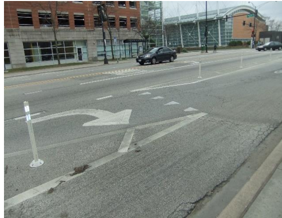
Figure 18: Right turn lane merging into bike lane, Chicago.
