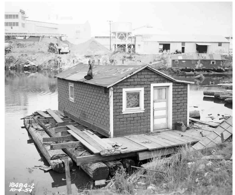
Figure 8: This home on the Duwamish river in 1954 is an example of the humbler (small and inexpensive) floating structures built during the Great Depression.
