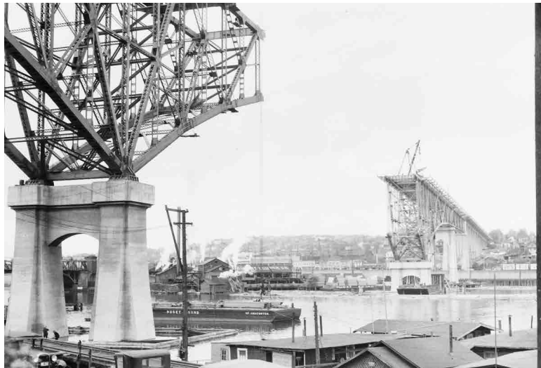
Figure 7: Floating Homes on Lake Union, 1931
