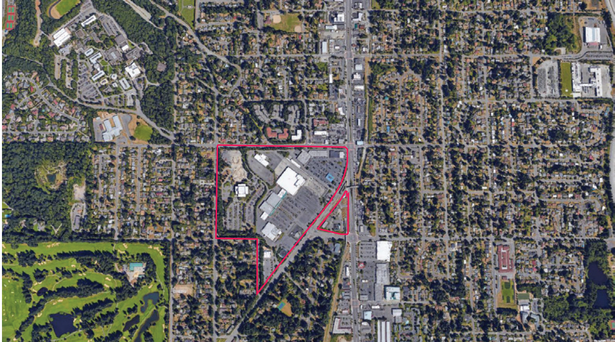
Figure 4.11 Aerial View of Aurora Square. Courtesy of: Google Earth
