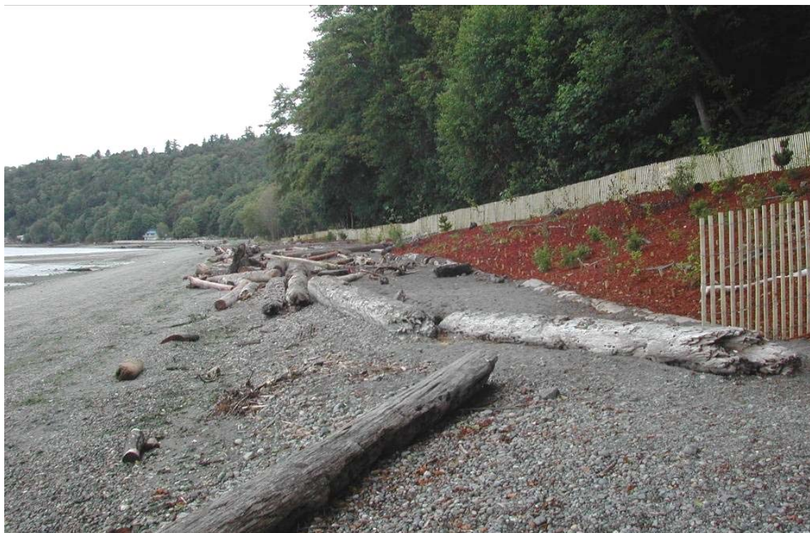
Figure 3. Restoration site after removal of the seawall.
