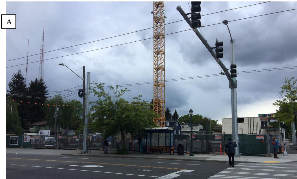
Figure 3.6 NW corner of 23rd & Union: Development in progress (Source: Author)
