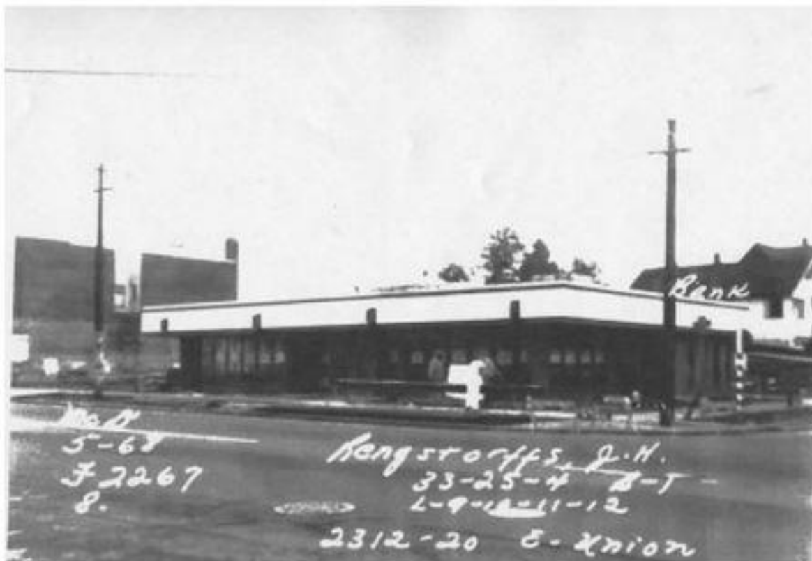
Figure 5.2 Liberty Bank in 1968 (Source: LibertyBankBuilding.org)
