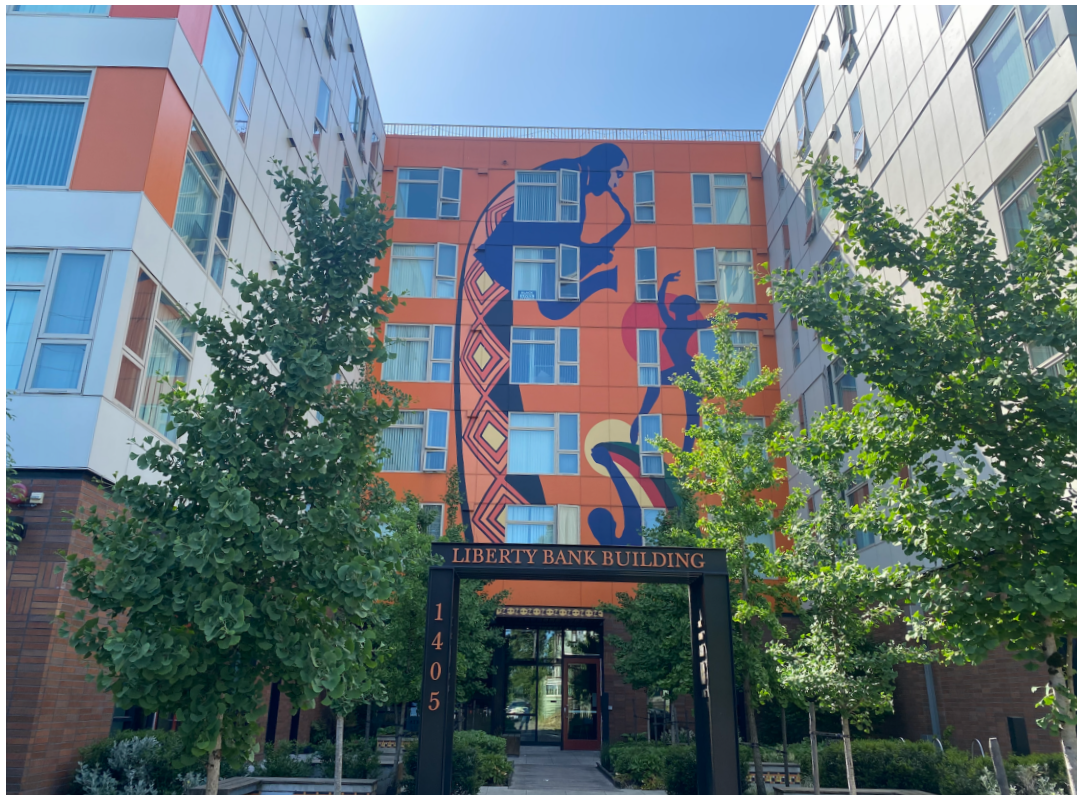
Figure 13: Liberty Bank Building Source: Personal Photograph (2023).
