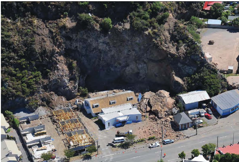
Figure 1.2: Large rock fall in Sumner, New Zealand (rock fall fatality reported at the building site left) [photo credit: GNS Science]
