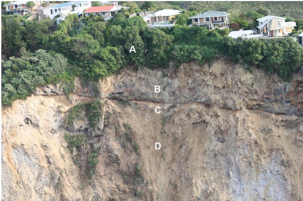
Figure 4.2: From Canterbury Earthquakes 2010/11 Port Hills Slope Stability: Debris avalanche risk assessment for Richmond Hill [71]: Geologic units at the Richmond Hill cliff face. A) Loess and fill covered by vegetation, B) Blocky columnar jointed basalt lava and breccia, C) Epiclastics, and D) Trachy basalt lava breccia.
