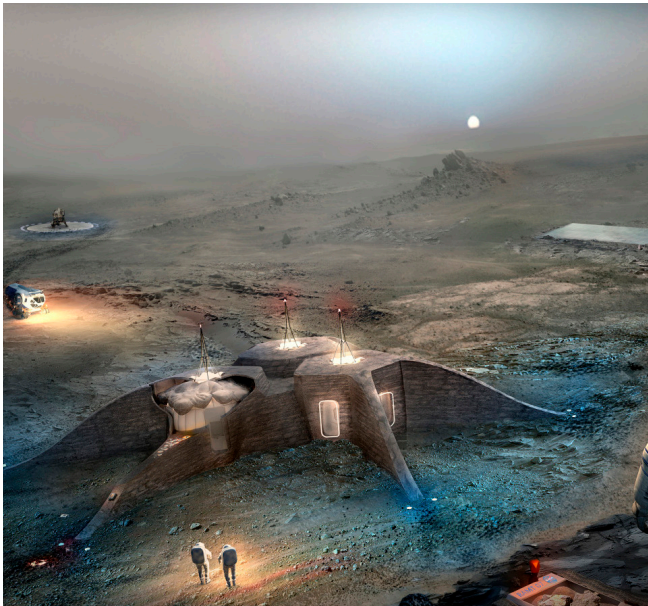
Figure 13: A proposed four-person habitat design that uses a pneumatic prefabricated core covered with mined Martian regolith. (Team Gamma/NASA, architectmagazine.com )
