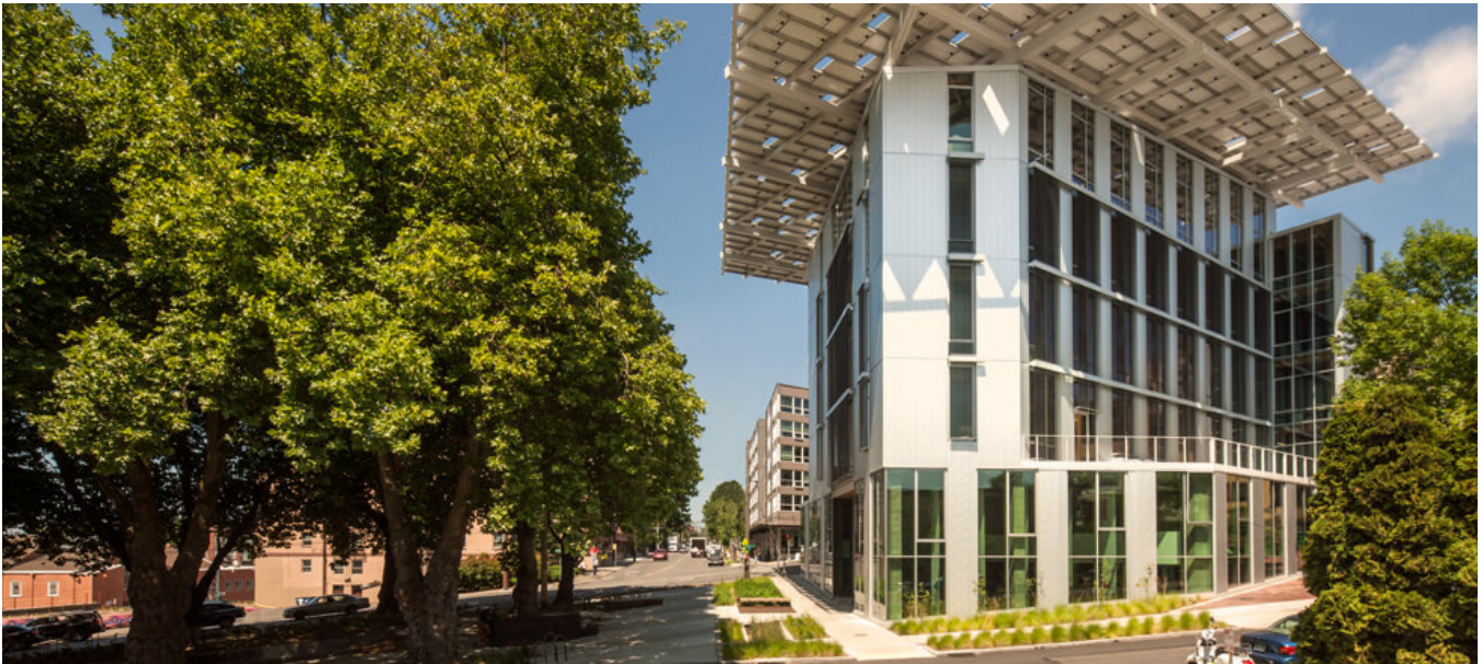
Figure 32: The Bullitt Center, Seattle. This “green” building exposes people to its functional systems through visible solar panels, plantings that filter stormwater, passive heating and cooling, and on-site waste treatment. (Bullitt Foundation, bullittcenter.org )
