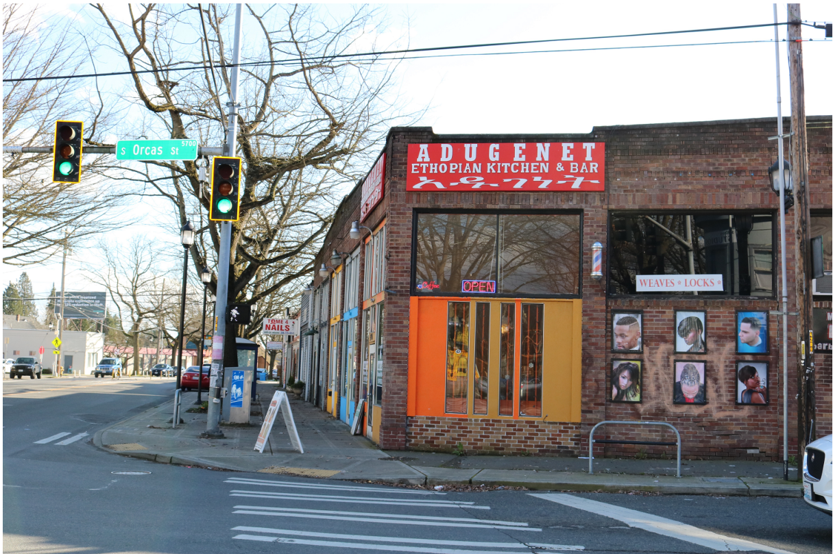
Figure 23: A typical Hillman City URM structure, Photo by Allen Medley (2018)
