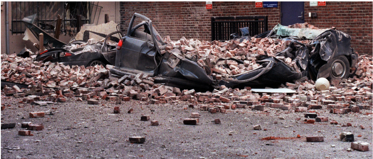
Figure 2: URM Collapse caused by Nisqually Earthquake (Seattle Post-Intelligencer 2001)
