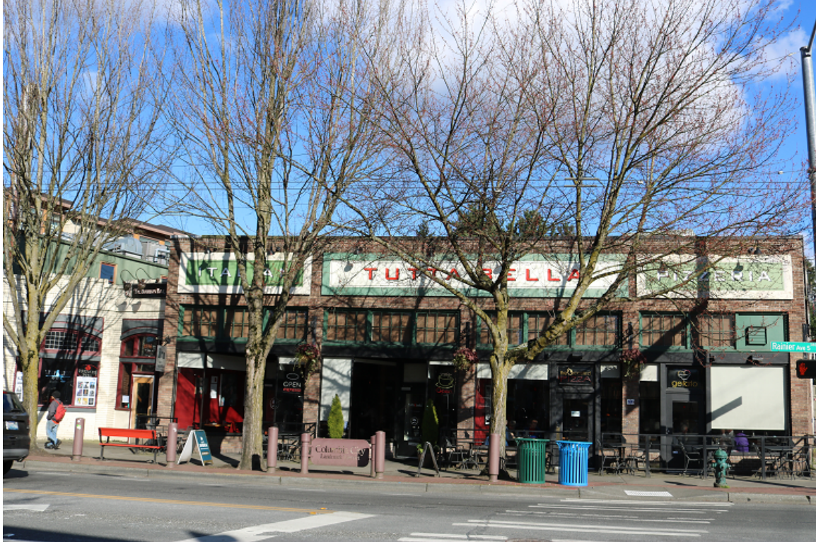
Figure 21: A typical Landmark District URM structure, Photo by Allen Medley (2018)
