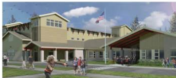
Ocosta elementary school built to also serve as a community vertical evacuation structure. Image from: www.oocosta.k12.wa.us
