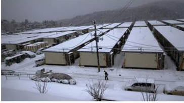
Temporary housing for Thousands of Families in Minamisanriku, Japan
