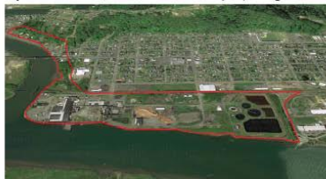
Aerial: Aberdeen and East Hoquiam, Washington The site is primarily located on an abandoned pulp plant
