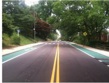
An example of high-visibility bike lane treatments. Accidents along this section were greatly decreased following implementation. Photo: City of Alexandria, VA
