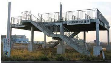
A tsunami refuge tower used in Yaizu, Japan. Photo source: https://upload.wikimedia.org/wikipedia/commons/thumb/7/77/777.jpg_20061121_Tsunami_Evacuation_Platform_001.JPG/1280px:777.jpg_20061121_Tsunami_Evacuation_Platform_001.JPG?1464900721289
