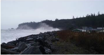
Seawall to protect the village of Taholah, WA from storm surges.
