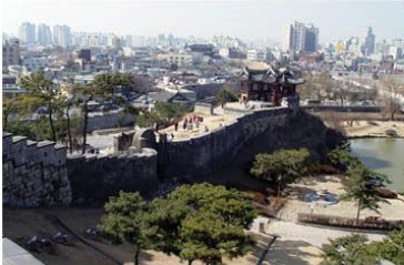
A section of the wall that runs through Suwon Korea. There is a pedestrian pathway on top of the wall surrounded by open space. Image from: Wikipedia.org
