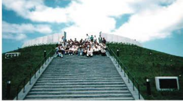
A berm constructed in Okushiri Island, Japan. Source: Tsunami Vertical Evacuation On The Washington Coast, Grays Harbor County
