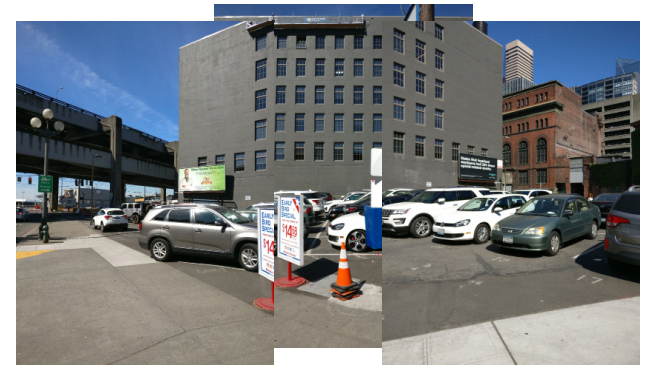
Figure 29 | On site, looking north at the south facade of the neighboring structure.
