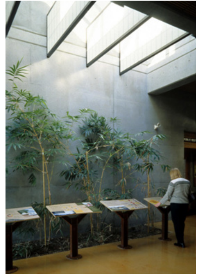
Figure 18 | The interior shear wall of the Pierce County Environmental Services Building with light washing.
