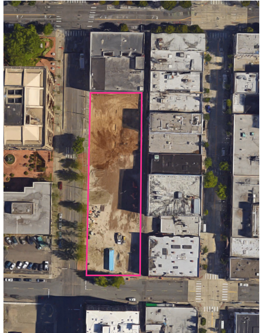
Fig. 51: Aerial of current site under construction.
