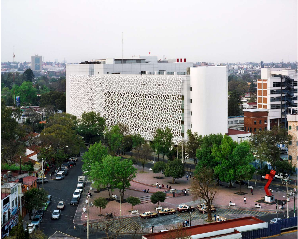
Figure 5. 2500m2 Facade at Torre de Especialidades, Mexico City. 2013 < http://www.prosolve370e.com/home >. Digital Image.
