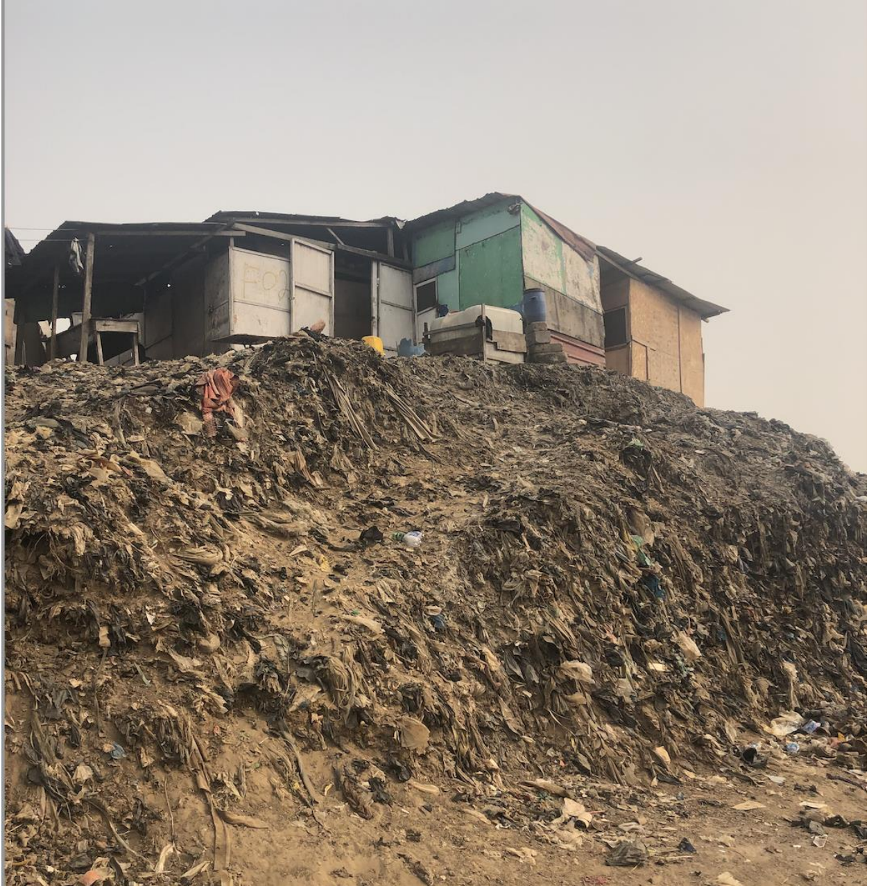
Figure 3.15: Another angle of the structure in Figure 3.14. This photo depicts a house in the Old Fadama informal settlement, Accra, which is built on top of a textile waste “mountain”. Photo taken by Ellie Cleasby on January 30th, 2024.
