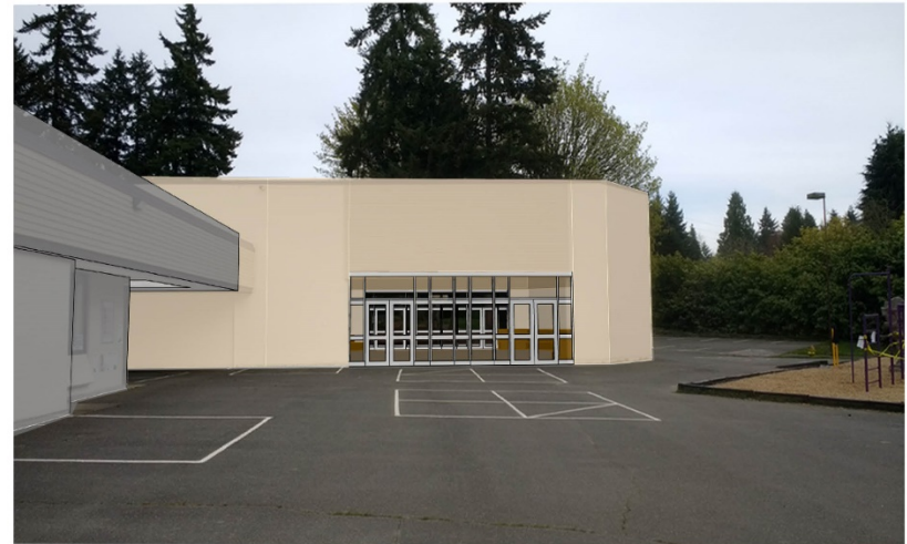
Figure 5.9. Views of the “quiet corner” alcove inside the proposed cafeteria addition for Rockwell Elementary.
