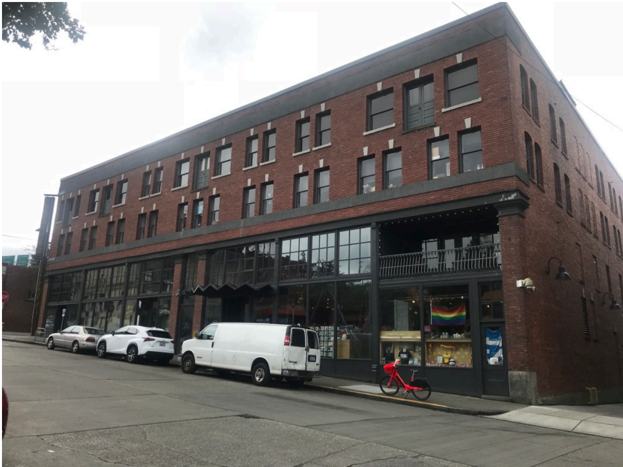
Figure 4: Kong Yick Building eastern façade (Source: Rachel Vickers, 2019)
