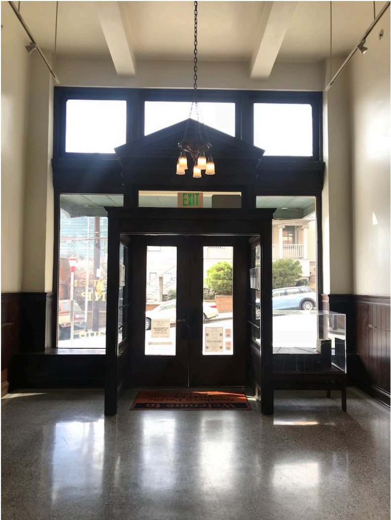
Figure 15: Lobby of NP Hotel. Steel K Bracing should be used near the windows of the lobby (Source: Rachel Vickers, 2019)
