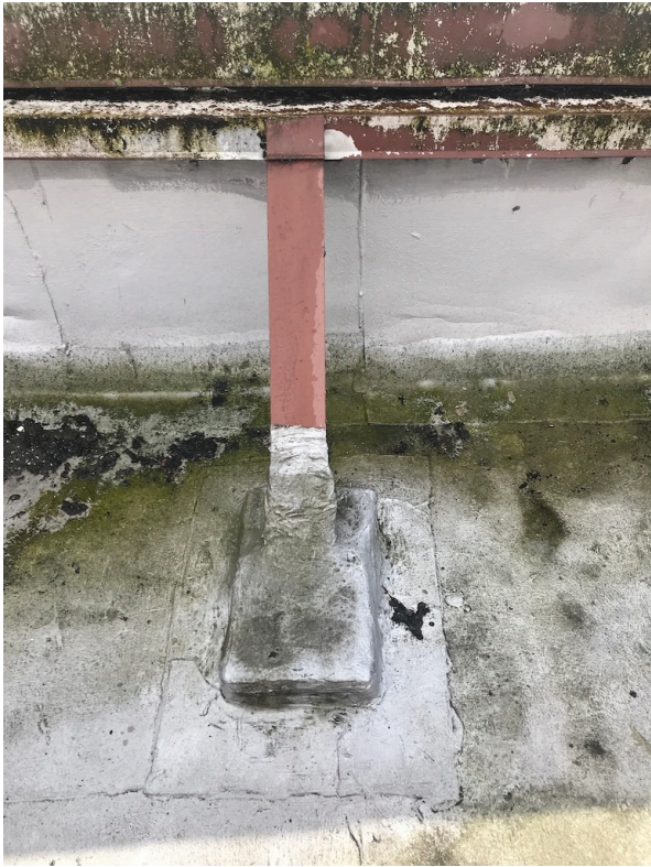
Figure 12: Parapet bracing on roof of NP Hotel (Source: Rachel Vickers, 2019)
