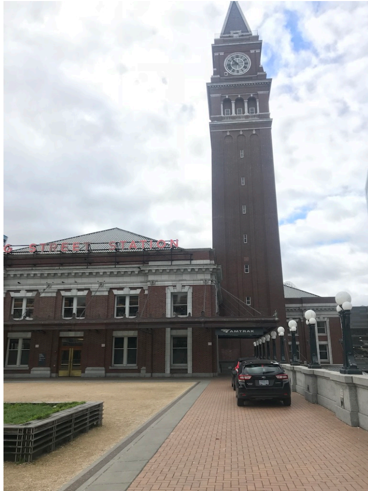
Figure 6: King Street Station northern façade and courtyard (Source: Rachel Vickers, 2019)
