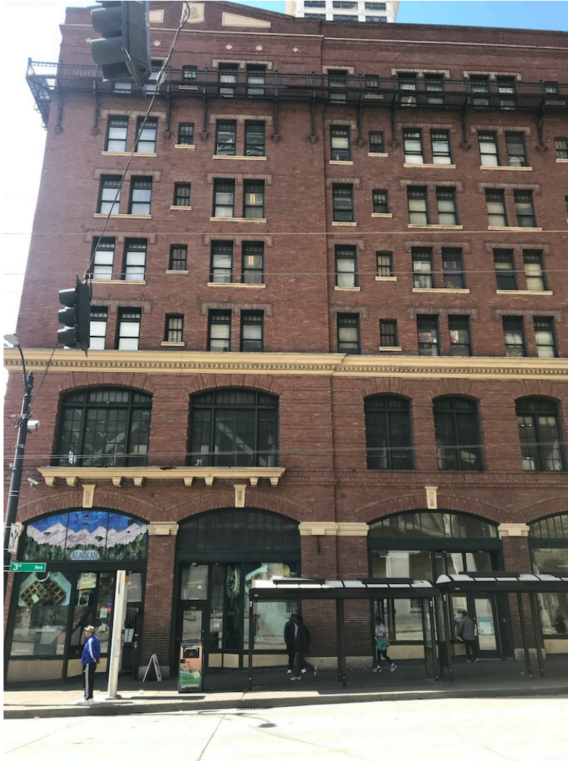
Figure 9: Detailed view of eastern façade of Morrison Hotel (Source: Rachel Vickers, 2019)
