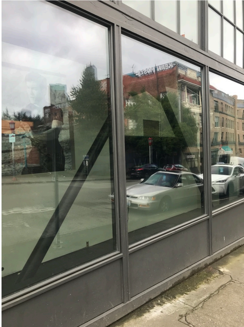
Figure 5: Interior Steel X bracing in Kong Yick buildings (Source: Rachel Vickers, 2019)
