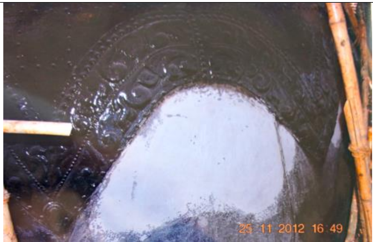
Figure 4.50. Brushing special glue before pasting gold leaf, showing the original decoration pattern of the pagoda.
