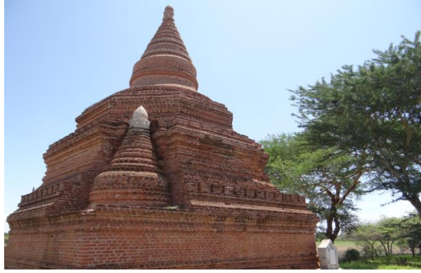
Figure 4.2. Encased pagoda and encased Buddha statue in Bagan. People found the inner layer after 1975 earthquake. Bagan Archaeology Office didn't restore the outer shape and leave it as it was to visitors.
