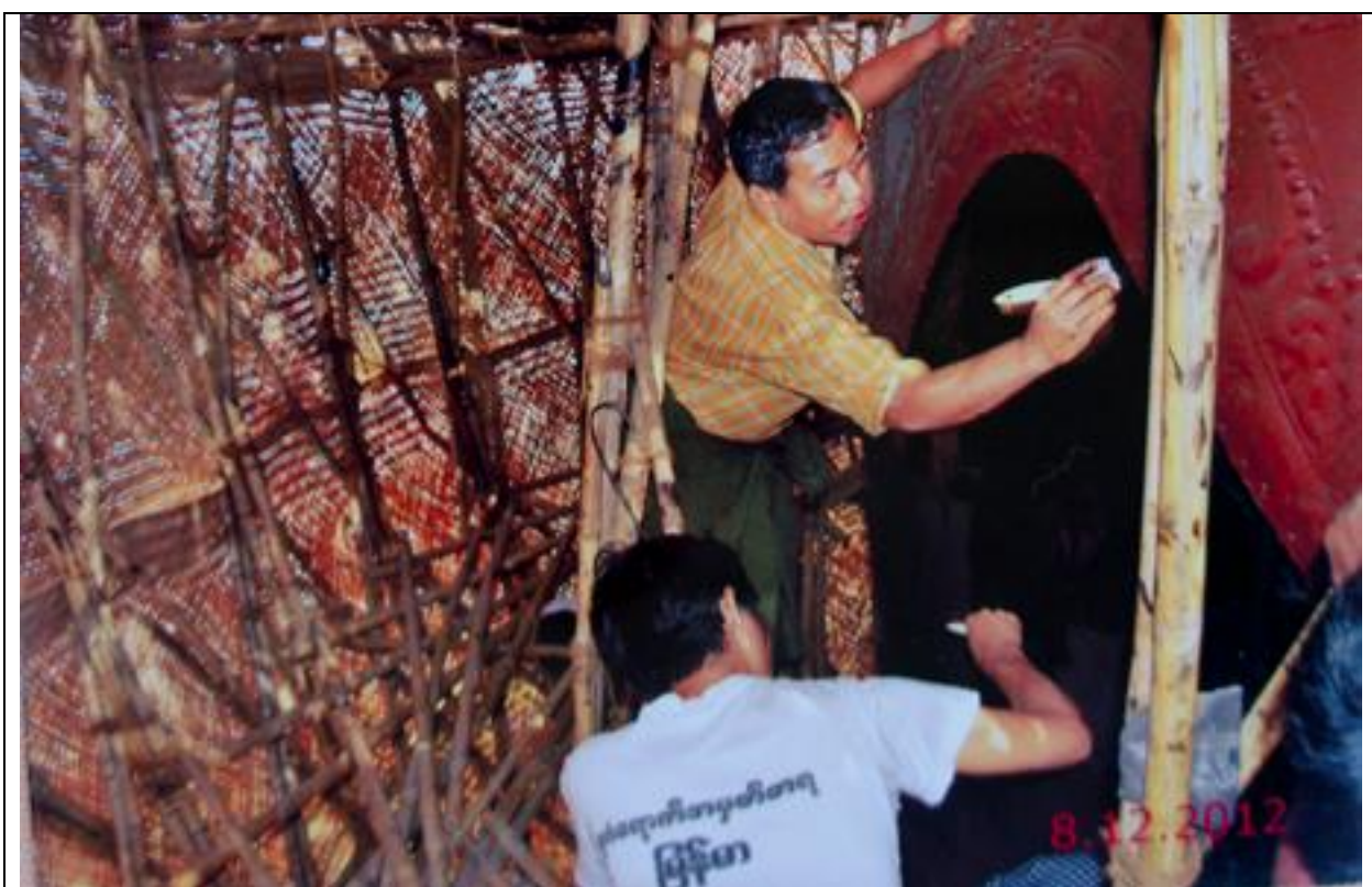
Figure 4.53 Brushing glue (the black color) before pasting gold leaf in the bell shape part of Bupaya.
