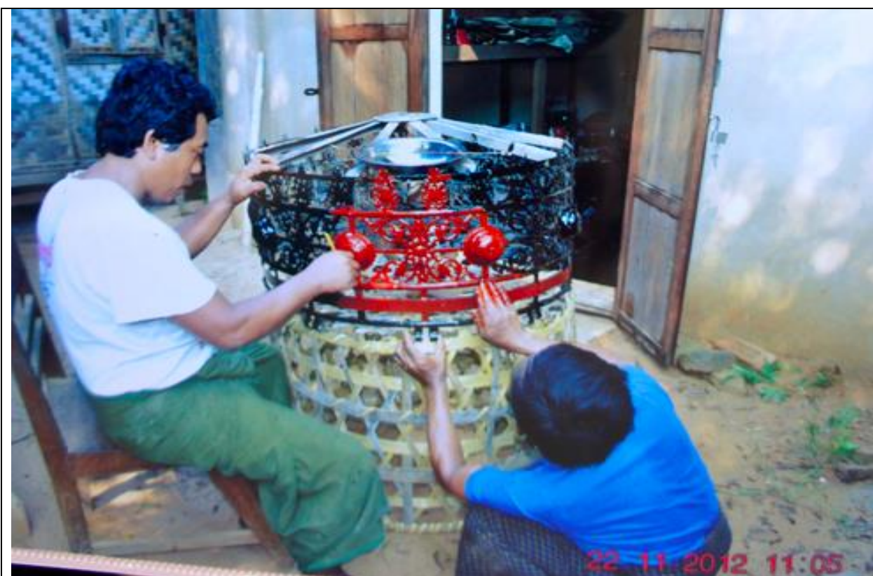
Figure 4.51 Repairing one layer of the Hti by local craftsman at the Bupaya Temple.
