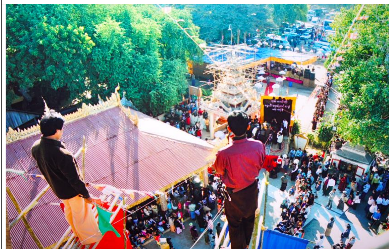
Figure 4.54 When workers finished gilding the pagoda, they would install the Hti at the top. View from the top of pagoda. Each part of Hti would be carried by the ropes we see in the photo.
