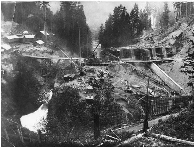
Figure 6: Construction of the Elwha Dam (Source: Nippon Paper Group)
