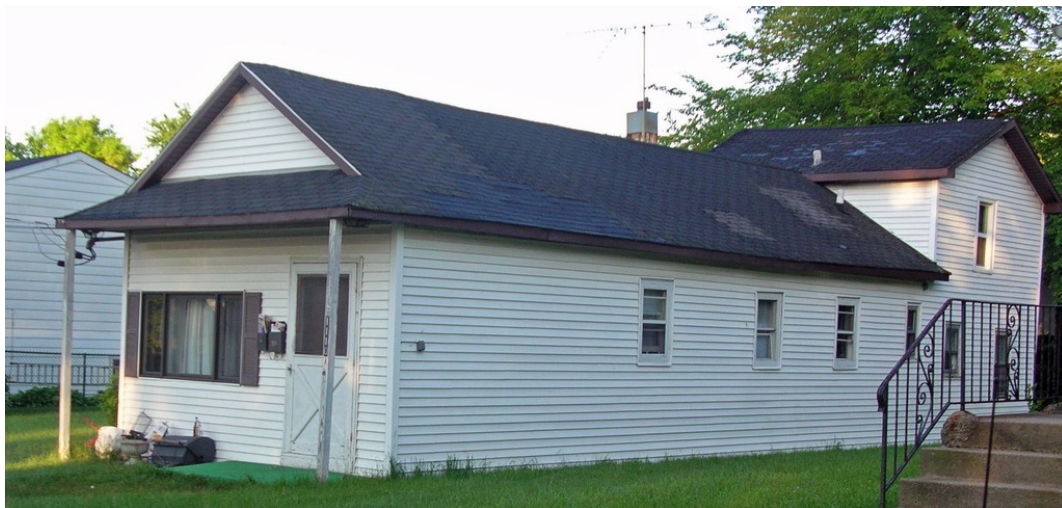
Figure 4 A home built by the tannery
