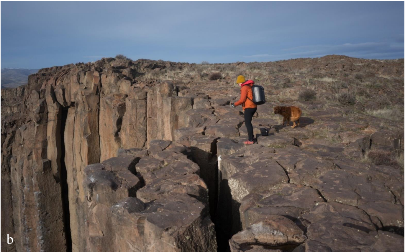
Figure 13: Column Separations. (a) Vertical aerial photo of the column tops near “Mr. Boshido” with people on the access trail at the foot of the wall. Note that separations appear larger closer to the face of the wall. This area had some of the smallest column separations. Scale bar is relevant to column tops. (b) Large column separation atop the routes Sunshine Buttrass and Mix it Up. This separation measures approximately 75 cm.
