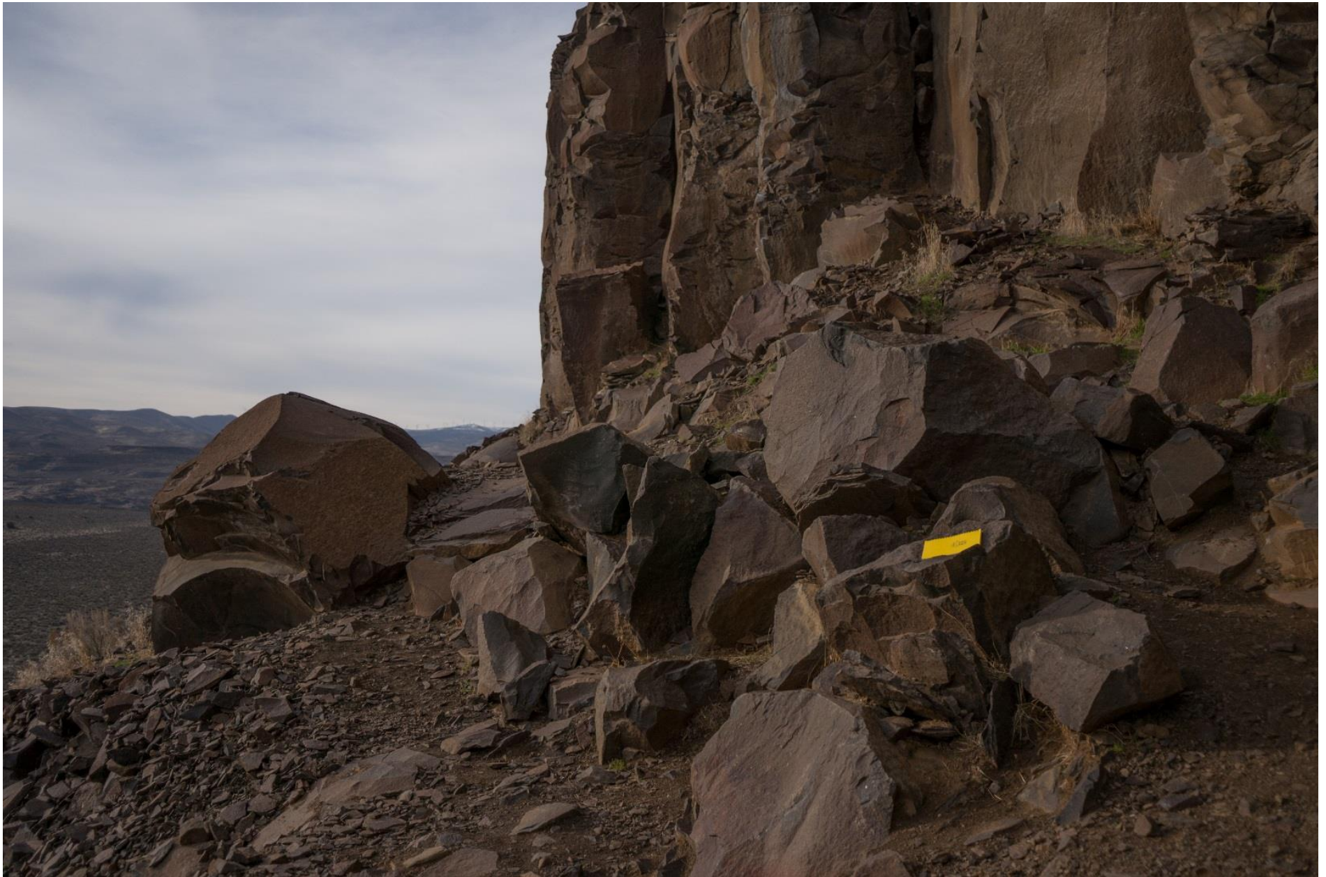
Figure 4: Column-sized debris at the base of the colonnade, Sunshine Wall. Image of the climbing trail at the western extent of the study area. Similar to the talus slope, large column sized blocks have accumulated at the base of the wall.
