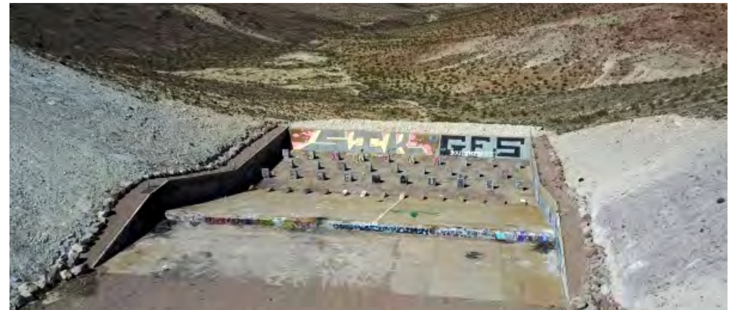
Figure 4.15. View of a typical detention basin used to store water and prevent flooding in the city. Image from the Center for Urban Land Use Interpretation.
