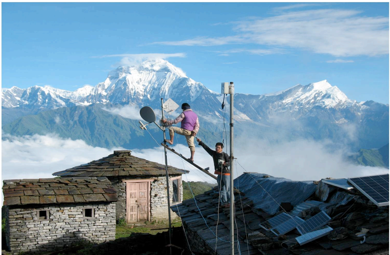
Source: Asia-Pacific Telecommunity: ICT Development
