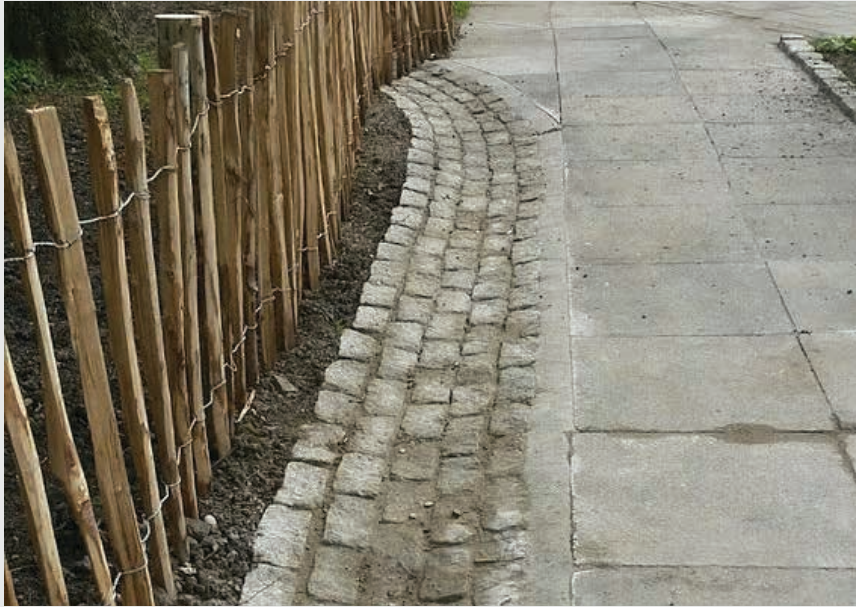
Figure 7.2: example of a brick runnel directing water into planting space (71)
