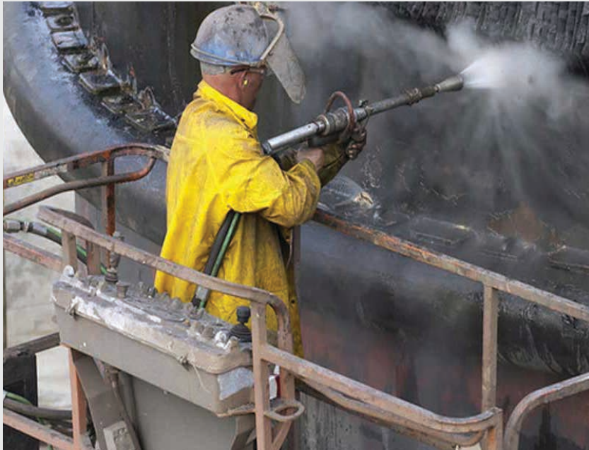
Figure 6.5: Industrial power washing can generally use nonpotable water (66)
