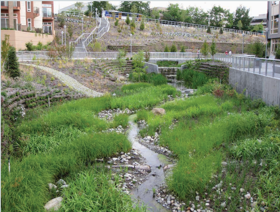
Figure 7.17: the Thornton Creek Water Quality Channel shortly after planting in 2009 (80)
