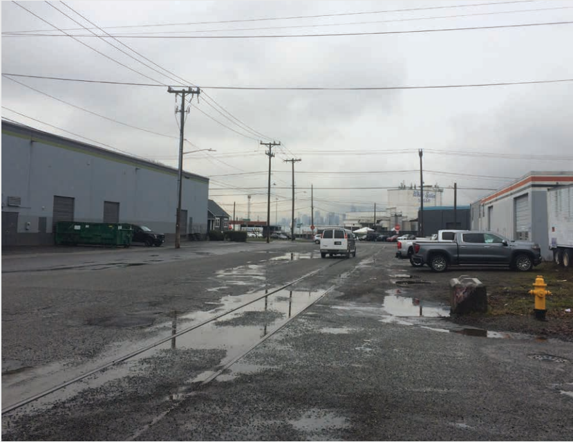
Figure 5.12: poor drainage conditions
