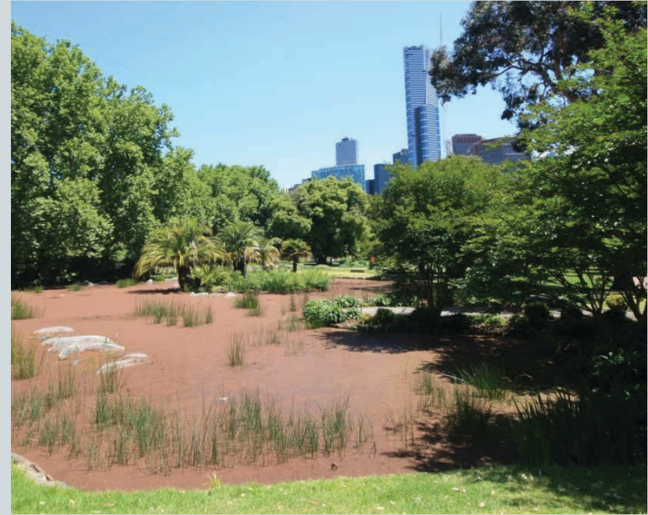
Figure 4.8: Dry stormwater storage pond at Queen Victoria Gardens in east Melbourne (33)
