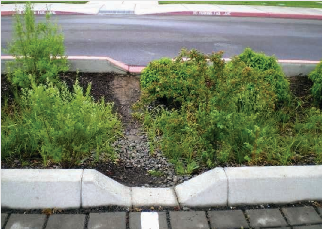
Figure 7.5: a purposefully poured curb cut that directs water into plantings (74)
