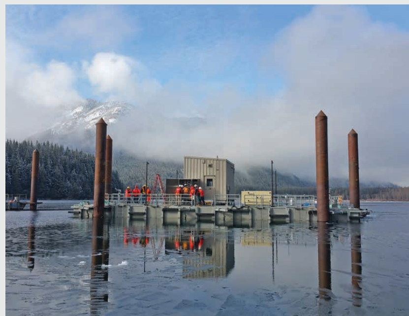
Figure 2.2: Morse Lake Pumping Plant (2)
