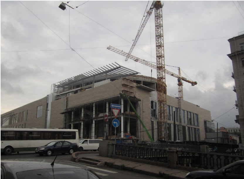
Fig. 55: Construction of Mariinsky Theater Second Stage, 2012
