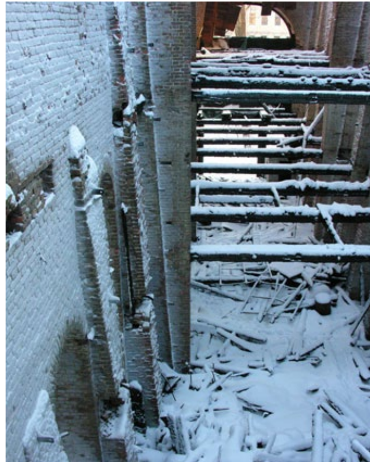
Fig. 21: View of the interior of New Holland Island's warehouses
