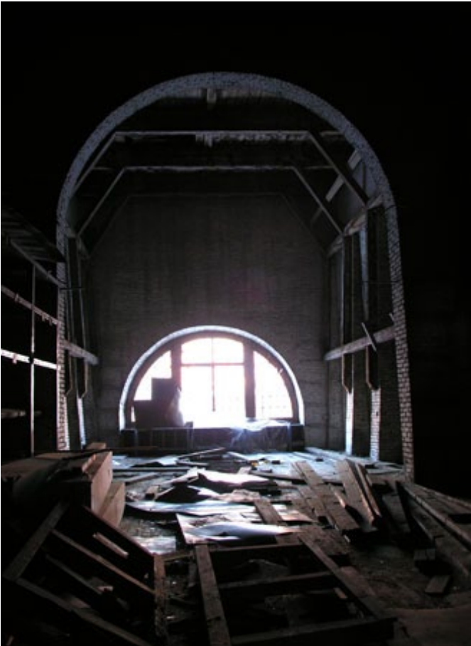
Fig. 20: View of the interior of New Holland Island's warehouses
