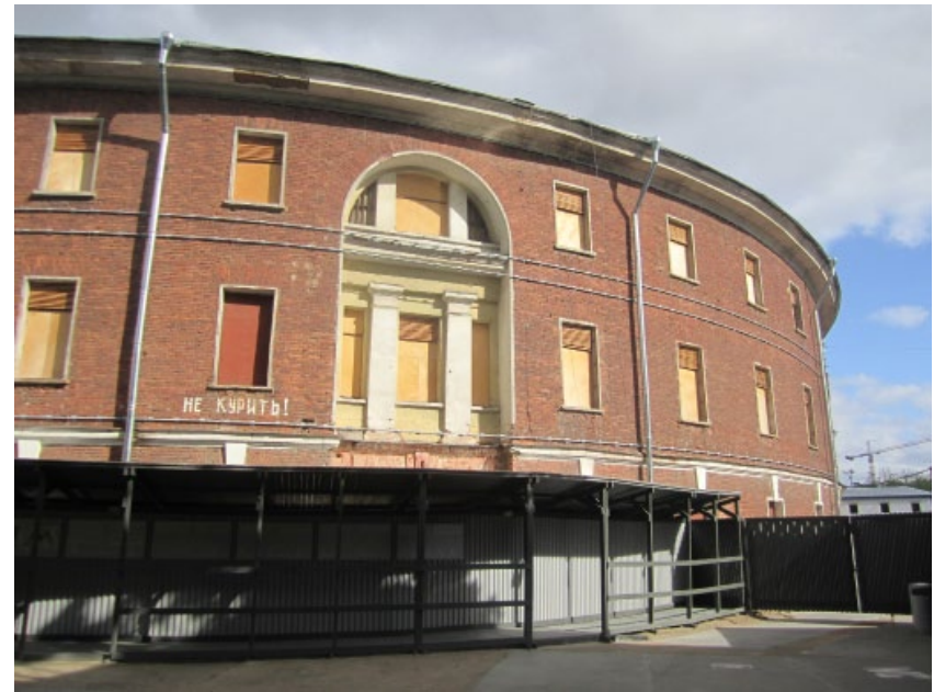
Fig. 17: View of the prison building today
