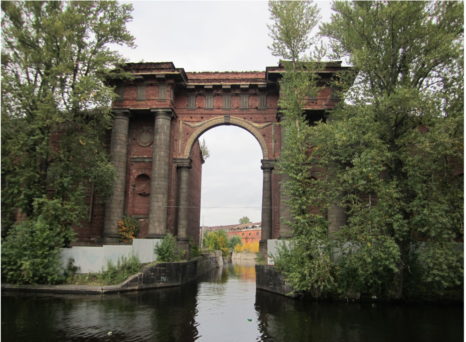
Fig. 52: View into the island under the archway
