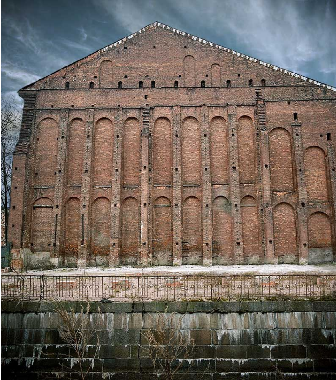
Fig. 44: End wall of warehouse structure
