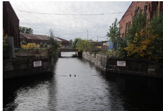
Fig. 40: View from Krukov Canal towards interior of the island
