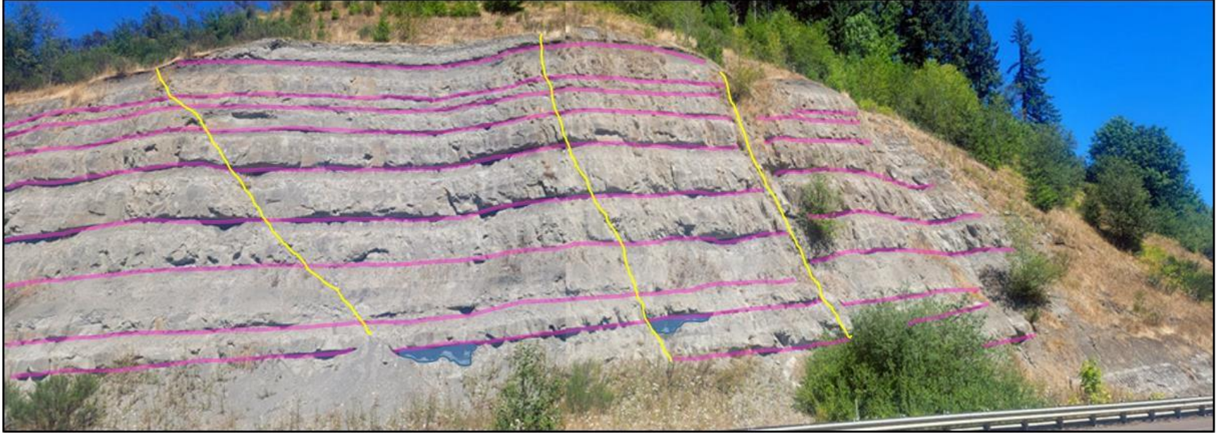
Figure 2.16 Eddyville, Oregon: major discontinuities (yellow) and water seepage areas (blue) in alternating beds of greywacke and siltstone (rose lines mark the bottom of each greywacke bed). Note that this image covers only the extreme east end of the site.
