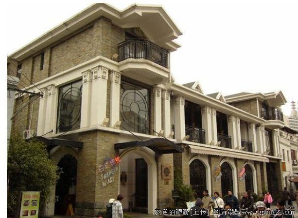
Figure 3.14 The renovated commercial building ( http://www.tplm123.com )
