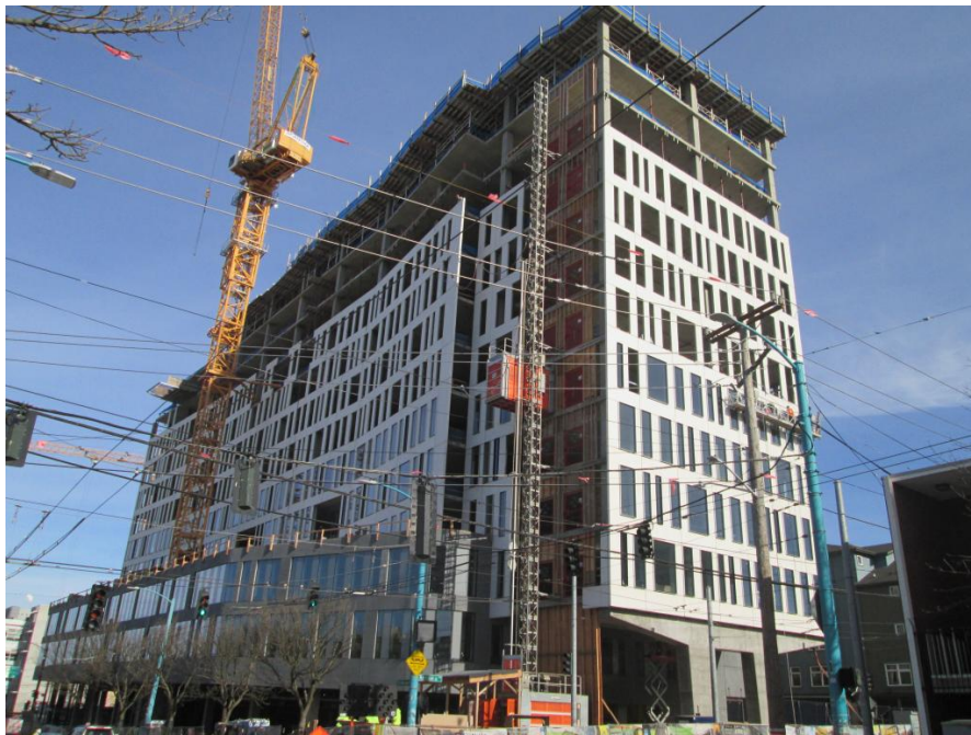
Fig. 7.1. Skanska’s 400 Fairview Project, February 2015.
