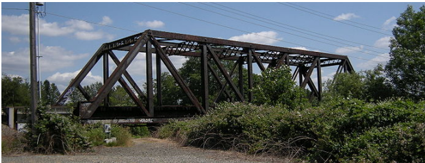
Figure 4.2. Truss Bridge from a neighborhood park
