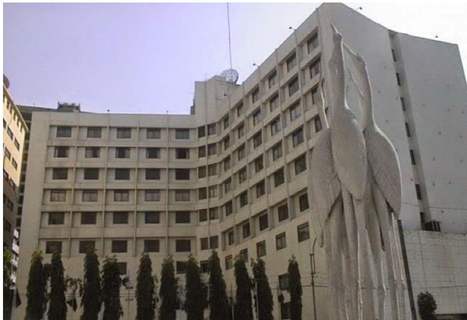
fig 29: Hotel Purbani, located in the Motijheel CBD area in Dhaka
