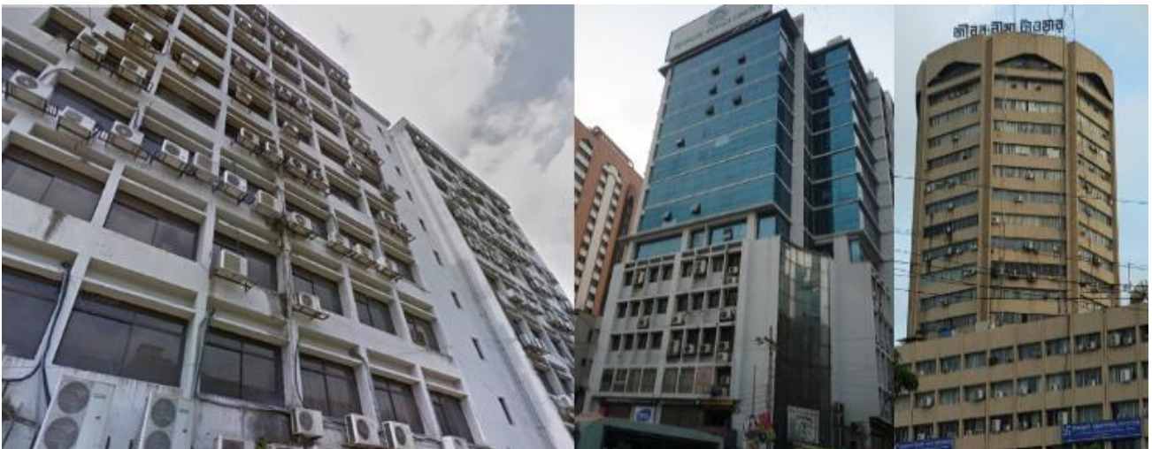
Fig 15: air conditioners and air cooler added on later to the high rises because of the artificially conditioned interior spaces
