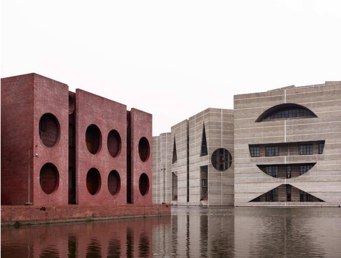
Figure 38: the parliament members' club with passive means of ventilation in red brick constructions
