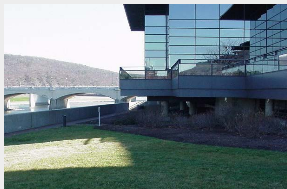
Figure 59: Elevated Pier Foundation . The facility is elevated on piers, allowing water to rise and flow under the first floor during a flood event (SCC 2016).
