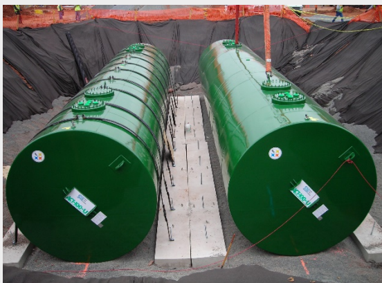
Image 74: Anchoring Fuel Tanks. Underground fuel tanks are being secured. Although underground, they could become buoyant in a flood (Tanks Direct 2015).
