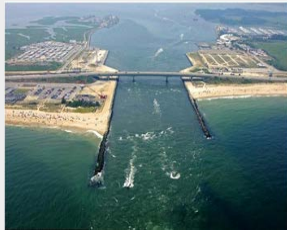
Figure 27: Harbor Entry . Groins are often used at the entry of a protected harbor or inland passage. They allow a strong delineated edge, which supports safe movement of ship and maritime traffic (Weebly 2016).
