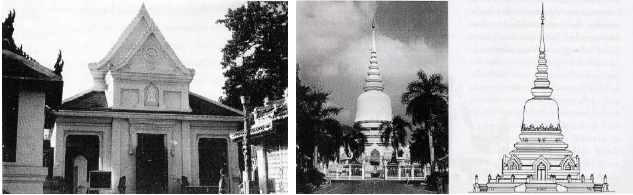
Figure 4-13 - Examples of the architectural concrete-structured style that based itself on traditional Thai elements: (left) the main building of Phra Pratom Chedi temple and the pagoda, built from concrete, at Wat Phra Sri Mahathat Woramahawihan, Bang Khen (right), Photograph, in Vimolsiddhi Horayangkura and el at., Pattanakan Naewkhwamkit lae Roopbaeb khong Ngansatapattayagum , [Development of Concepts, and Architectural Patterns: Past, Present, and Future] (Bangkok: The Association of Siamese Architecture, 1993), 86 and 91.
