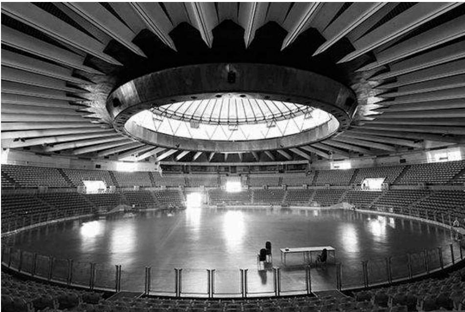
Figure 2-8 – The interior of the Indoor Stadium at Hua Mak, Photograph by Beer Singnoi, “Indoor Stadium Hua Mak, designed by Louis Bergers Company since 1966” SCG Experience , accessed March 14, 2022. https://www.pinterest.com/pin/454230312388406497/
