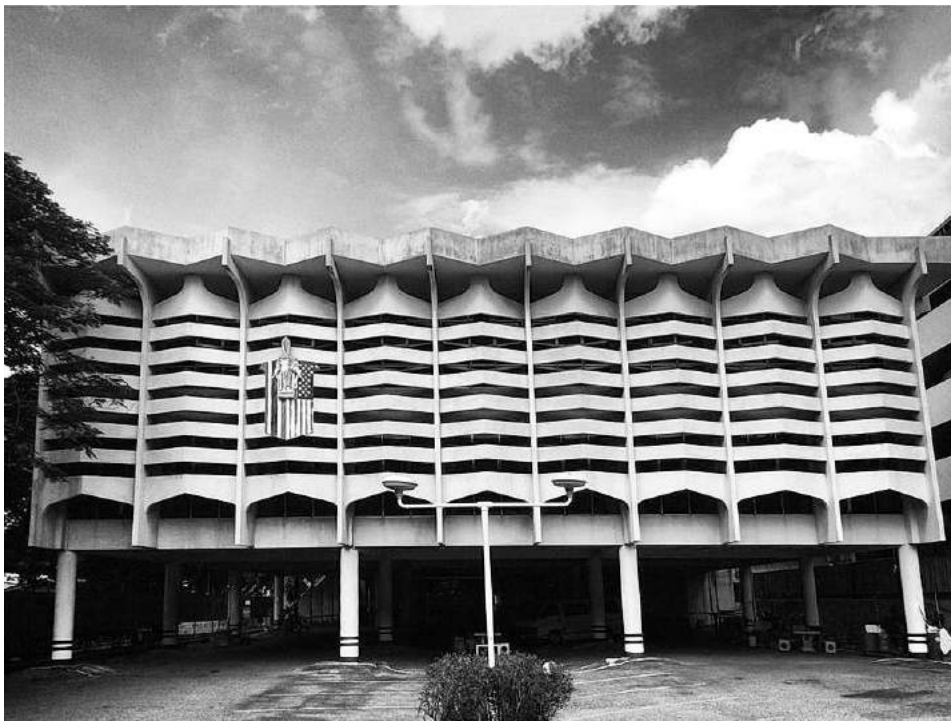
Figure 3-18 - Krisda Arunvongse's concrete-fin brise-soleil technique that was used with the American University Alumni building, Photograph by Beer Singnoi, "100 Amazing Architecture with SCG 100th Year Anniversary" SCG Experience , accessed March 15, 2022.
