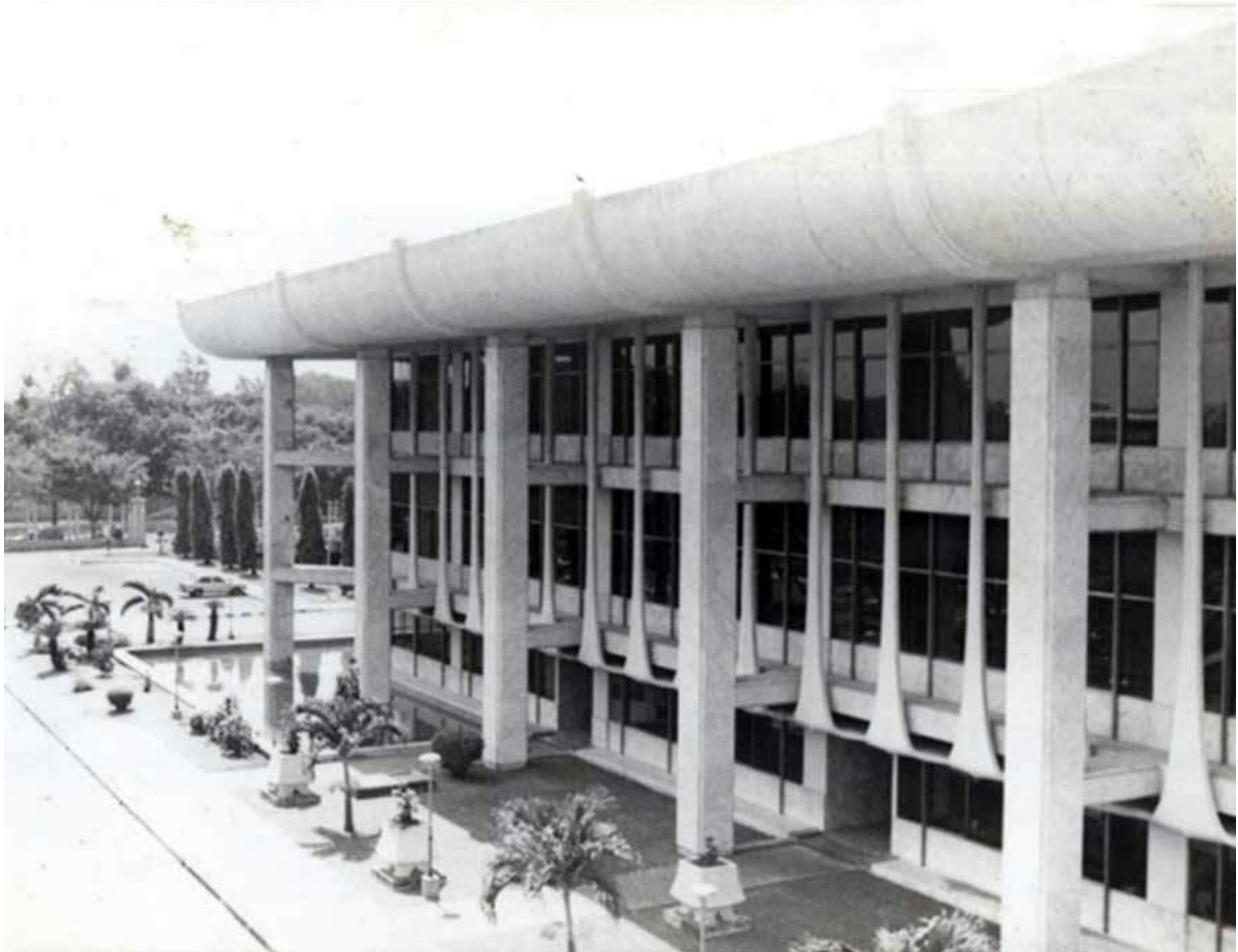
Figure 4-29 - The design component that vividly recalls Le Corbusier’s design to the utmost are the curved parapet and the concrete piers that wrapped around the building, Photograph, from “Pien-pan Rattasapha Thai” [The Changes of Thai Parliament Buildings], Parliamentmuseum.go.th , June 28, 2021, https://parliamentmuseum.go.th/89y/content4.html
