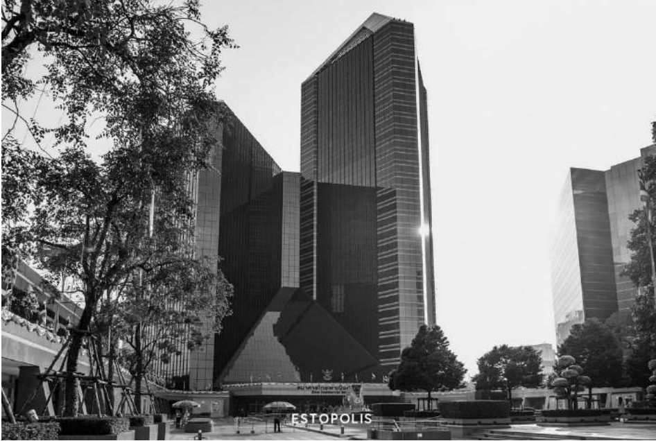
Figure 2-13 - The overall complex of SCB's headquarters, Photograph by Estopolis, "SCB Park Plaza," Estopolis , accessed March 14, 2022. https://www.estopolis.com/
