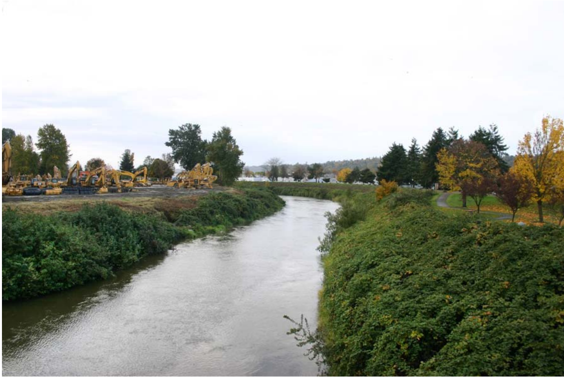
Figure 1-8. Most reaches of LGR are lined with overly-steepened levees and revetments that are covered predominately by Himalayan blackberry ( Rubus discolor ) and invasive knotweed ( Polygonum spp.) (WRIA9 Implementation Technical Committee 2012). The photo shows a reach confined by a levee to the right and a revetment to the left.
