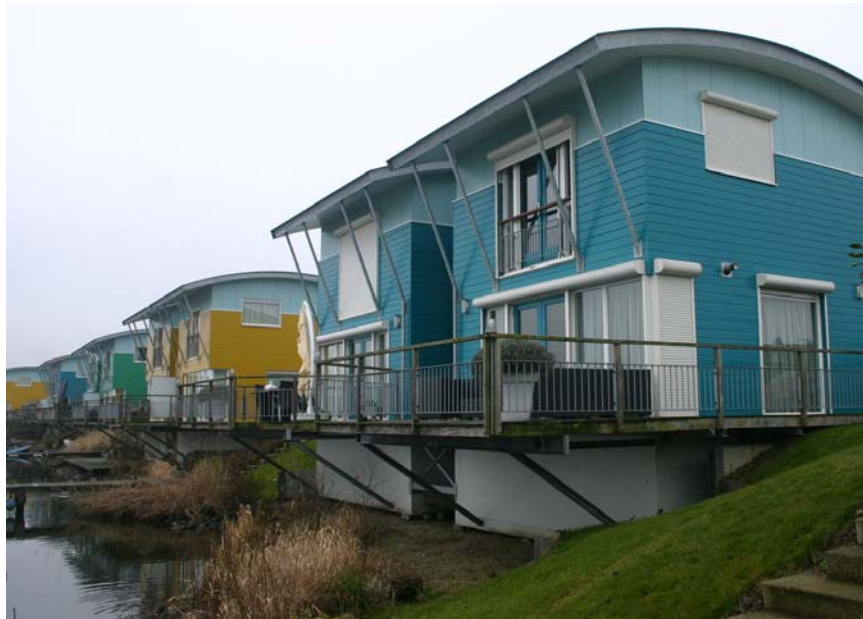
Figure 3-4. Amphibious houses in Maasbommel, the Netherlands. They are built on dry land but capable of floating during flooding because of the concrete box foundation that gives the house buoyancy. Photo credit: Kuei-Hsien Liao.
