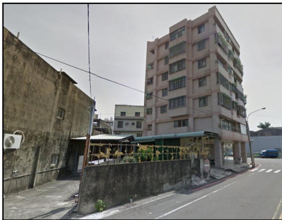
(a) East Face of Structure
