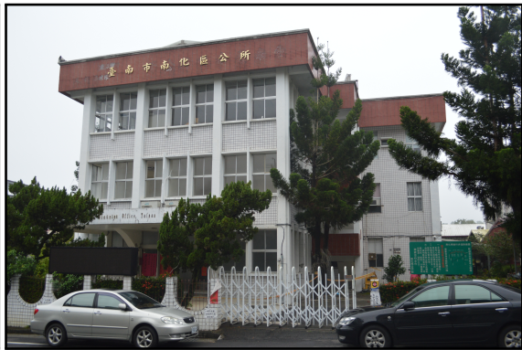
(b) East Face of Structure
