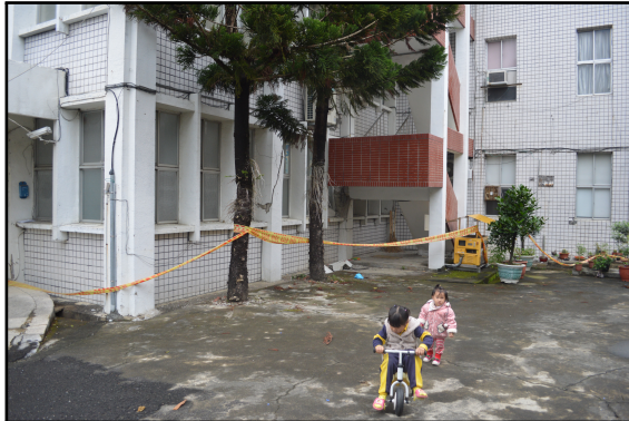
(c) Stair and North Side Bump-out of Structure
