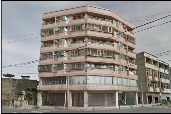
(a) North and West Faces of Structure
