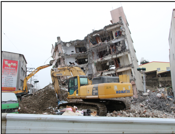
(c) Visible Tilt of the Structure (West to East) During Demolition
