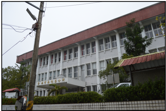
(a) South Face of Structure
