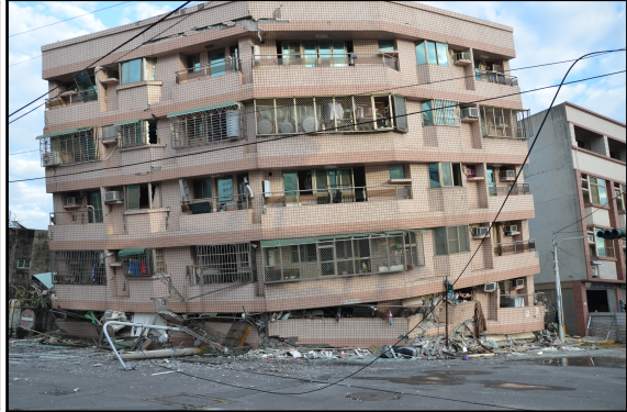
(b) Collapse, Crushing Stories 1 and 2
