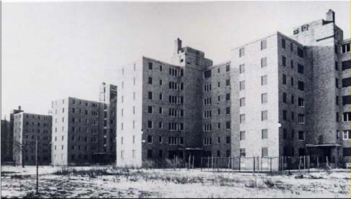
Image 11: "Columbia Point before its redevelopment"
