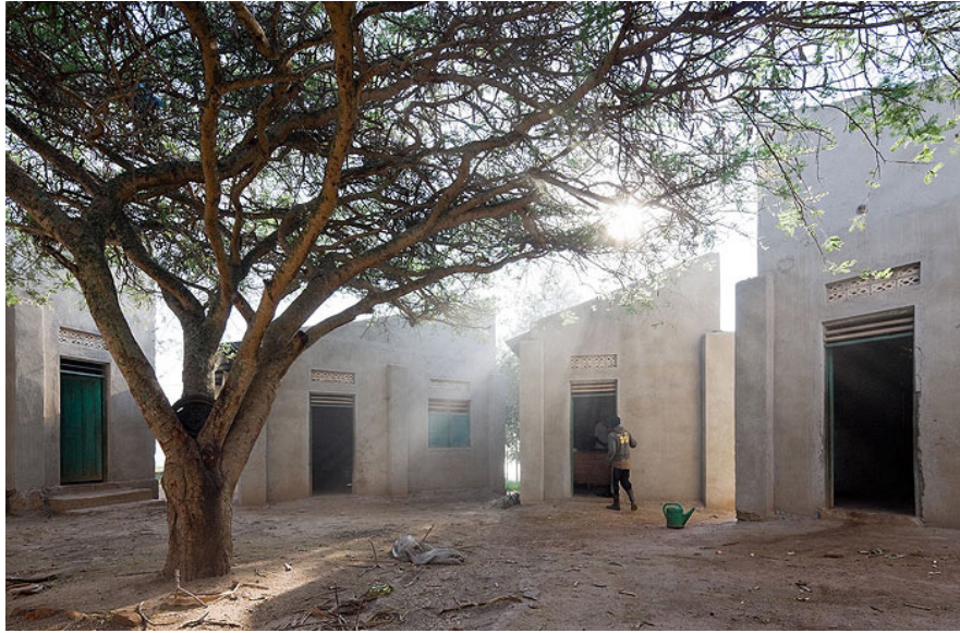
50 Courtyard Surrounded by Structures
