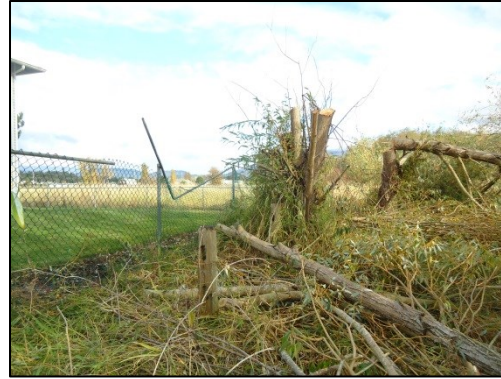
Photo 8: Broken mitigation area fence (wood) with adjacent property's fence (metal) damaged from fallen mitigation area tree
