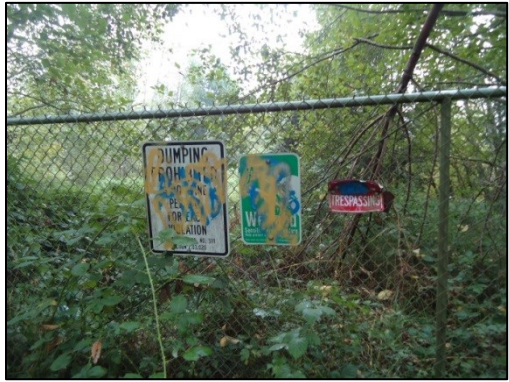
Photo 6: Graffiti on wetland protection area signage and wildlife barrier fencing
