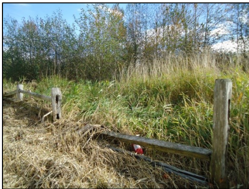
Photo 3: Broken fence and garbage
