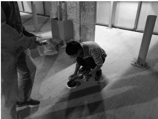
(a) Installation Process
