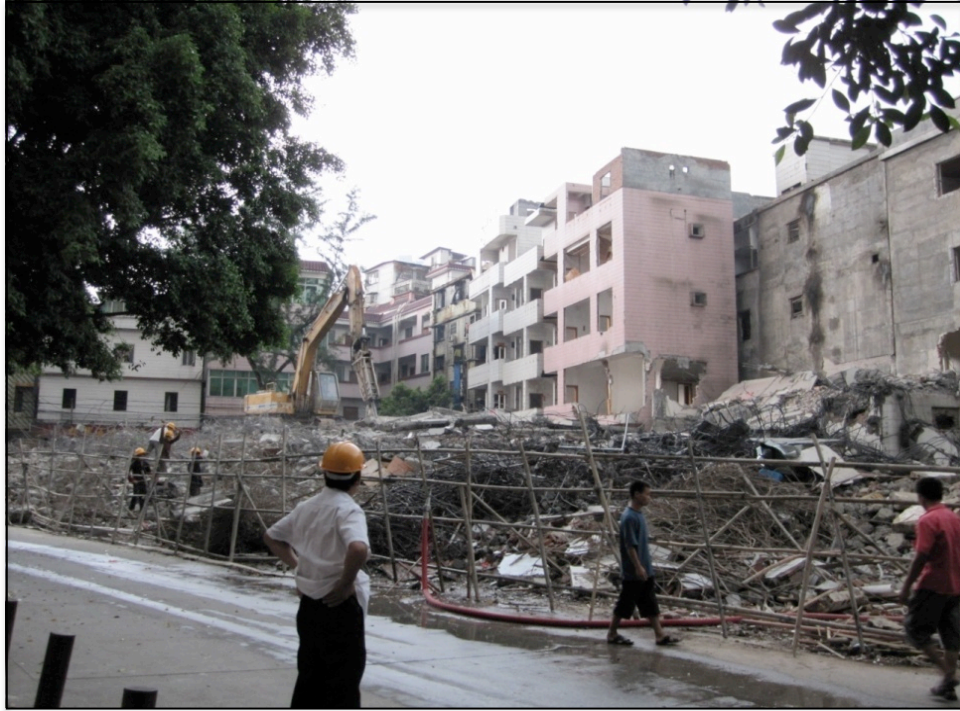
Figure 5.6 Yangji under Demolition (Source: photograph by the author in September 2010)
