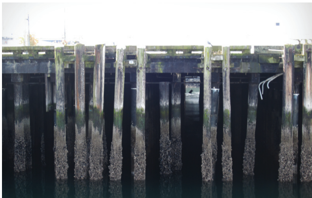
Pier 48's existing structure is deemed unsafe for reuse and any use of the property would require new building
