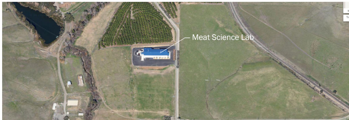
2.16 The J and G Lau Meat Processing Center, Cal Poly, Aerial View
