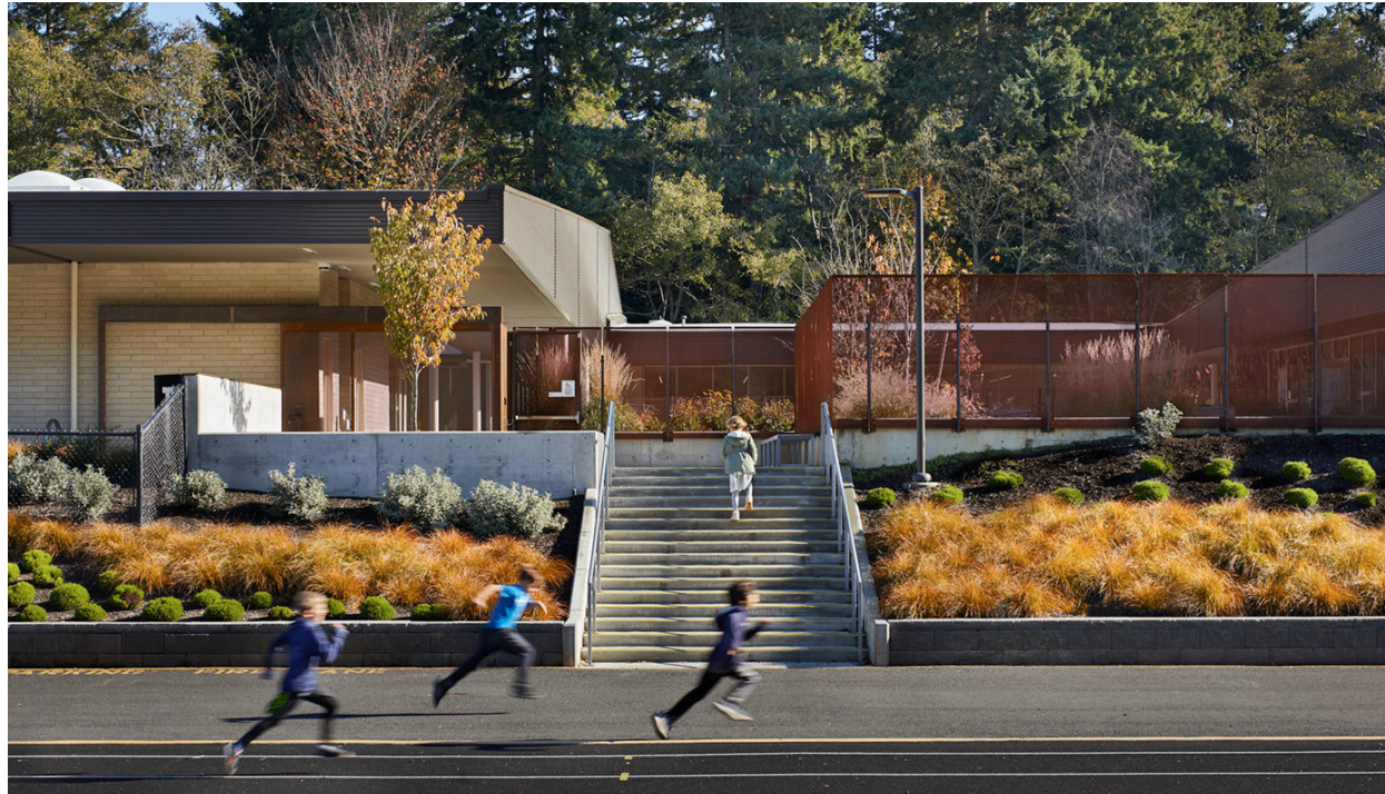
Figure 3.10 : Madrona K-8 School Building Exterior. Image from Forma Construction.
