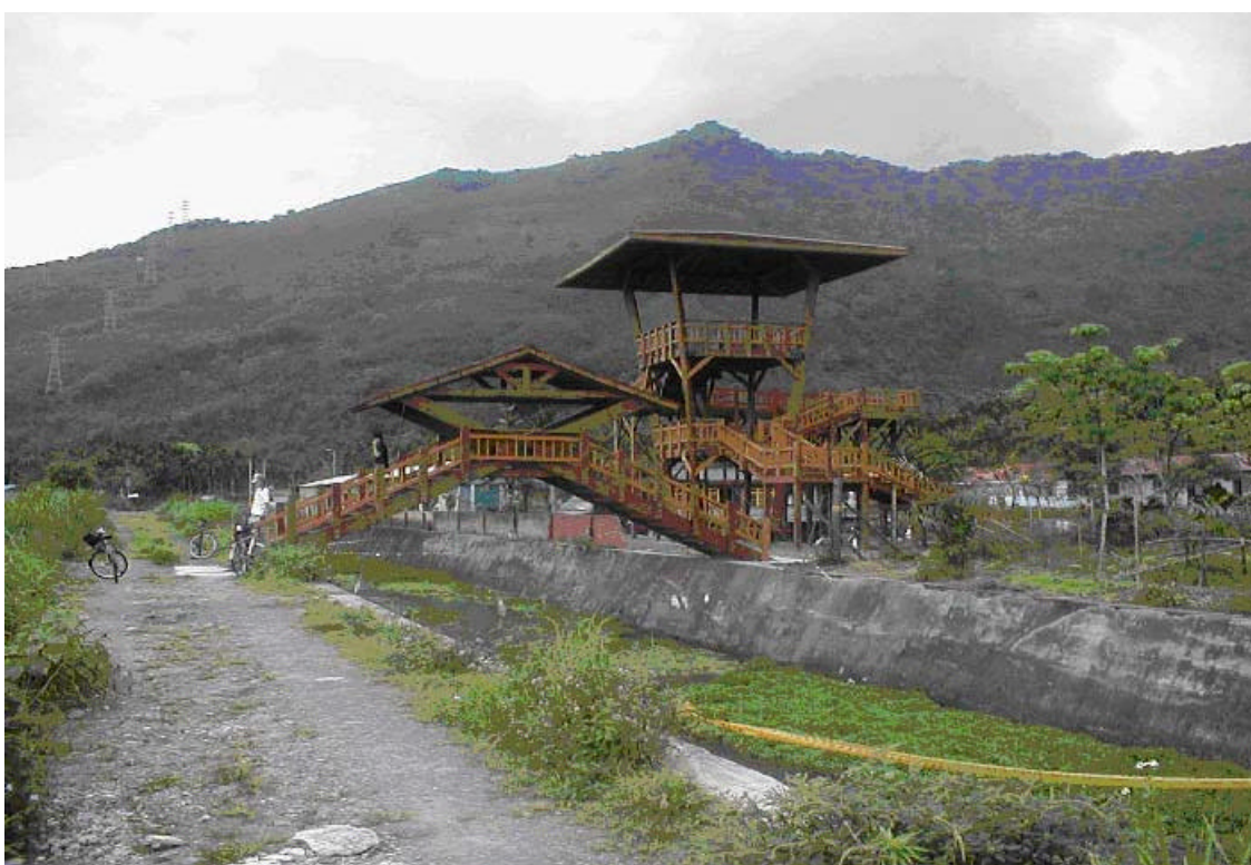
Photo 2. Wooden Viewing Platform Constructed of Treated Southern Yellow Pine Lumber at an Aboriginal Development near Hualien.
