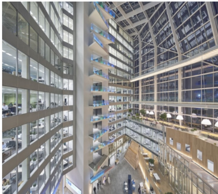
Fig.6: Atrium 15 story is big source of Daylight harvesting
