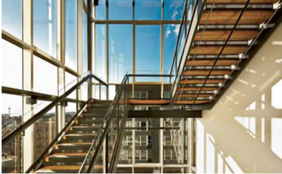
Fig.2: Bullitt Center staircase
