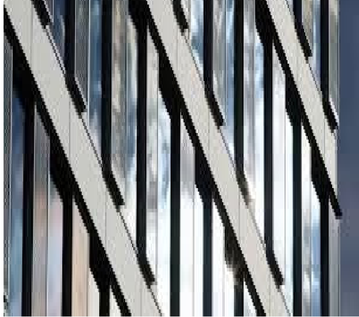
Fig.5. BIPV cladded with concrete on 40% of south facade
