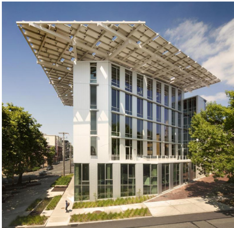
Fig.1. Bullitt Center with extended roof line with BIPV
