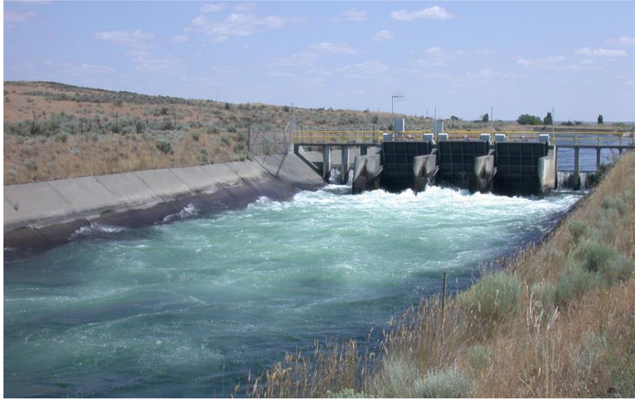
Figure 1.3-High Hills gates in the West Canal located in Columbia River Irrigation District. (Photo: Courtesy of Professor Philip Malte)
