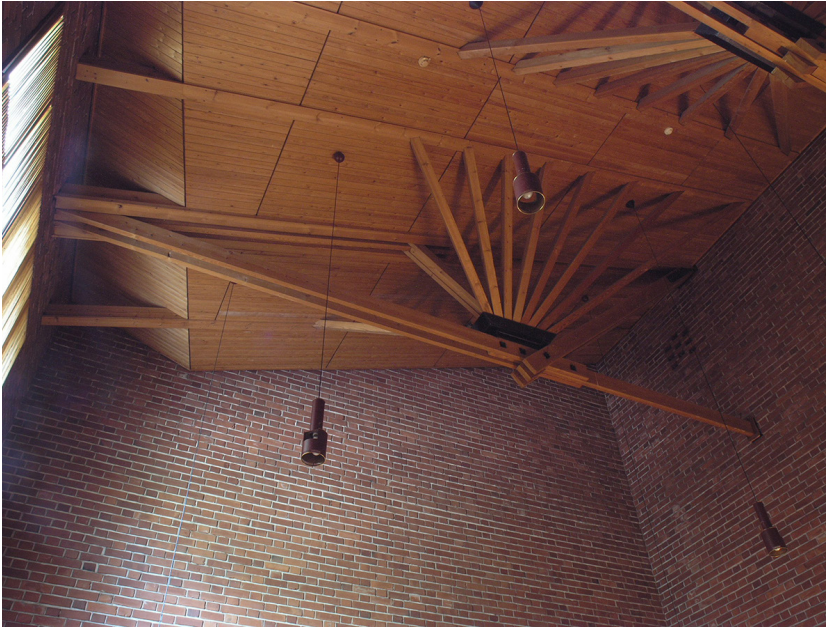
Above: Figure 32. Ceiling wood beams and trusses of inner council hall.
