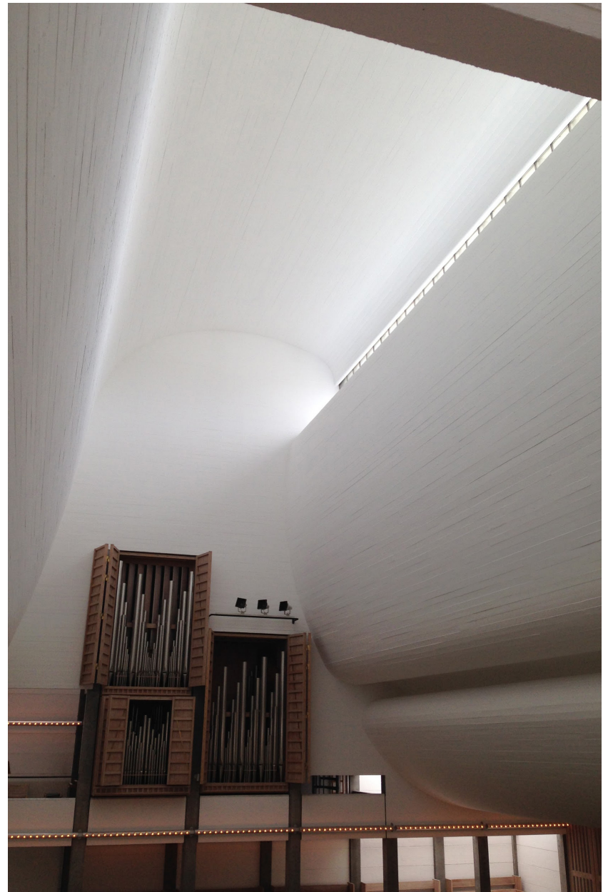
Figure 42. Curving concrete walls bring the light from the clerestory windows down toward the altar.
