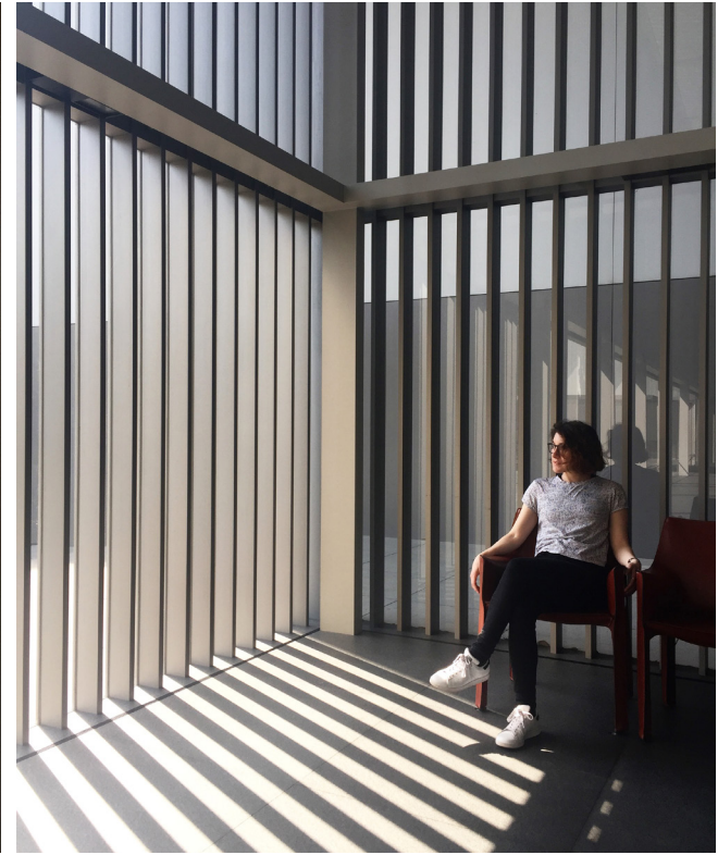
Figure 31. Sunlight is filtered through structural mullions in the double-height foyer.
