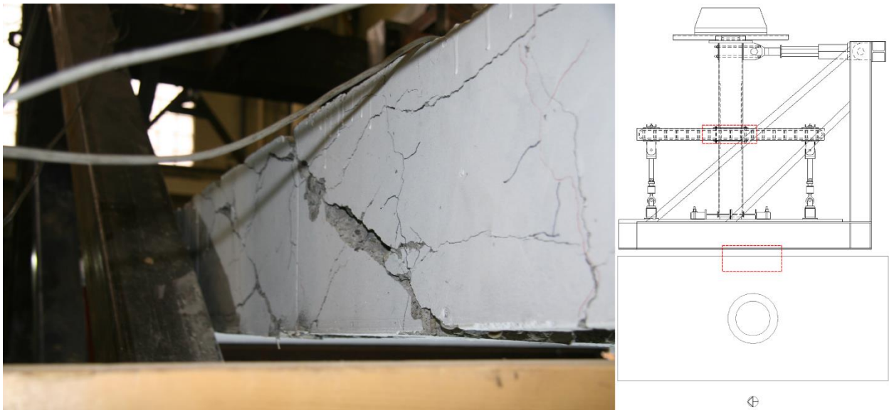
Figure 4-46: East Edge Shear Cracks – 4.8% Drift (PTB_4.5_1_0)
