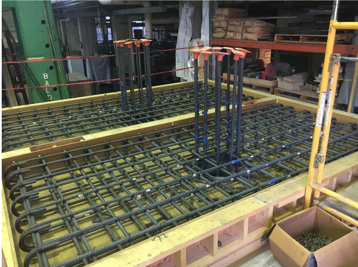
Figure 3-9: Completed Rebar Cage for Specimens PTB_4.5_1_0 and PTB_4.5_1_4
