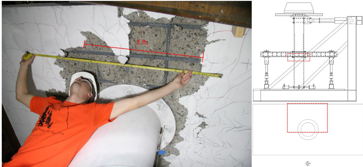
Figure 4-44: Bottom East Side Concrete Crushing – 4.8% Drift (PTB_4.5_1_0)
