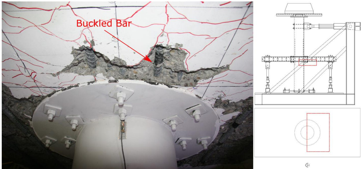
Figure 4-92: Bottom South Side Bar Buckling – 6.4% Drift (PTB_9_2_0)
