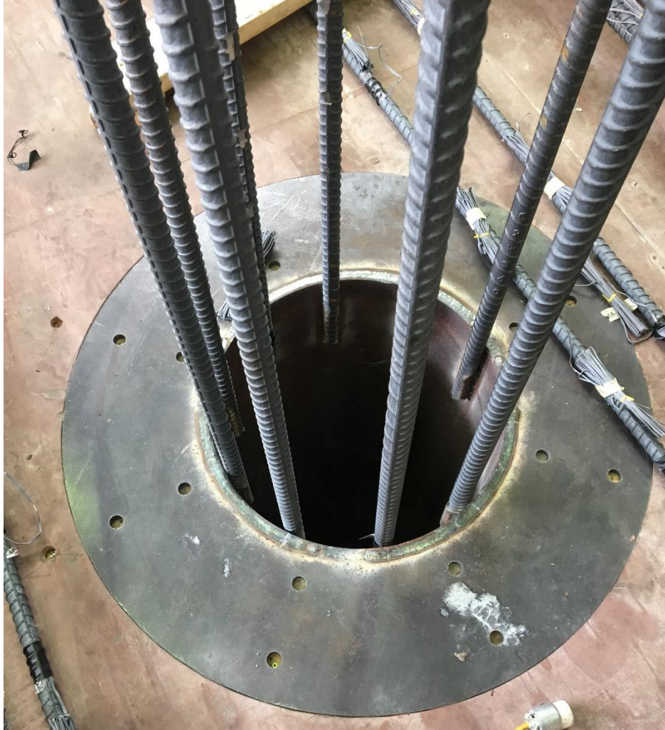
Figure 3-8: Welded Ring-Tube-Reinforcing Bar Placed in Slab Forms
