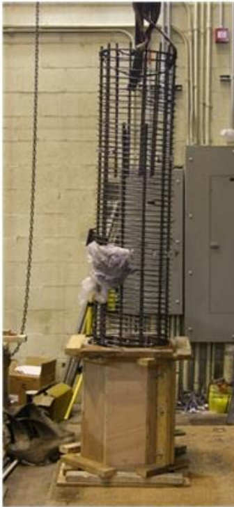
a). Column reinforcement
