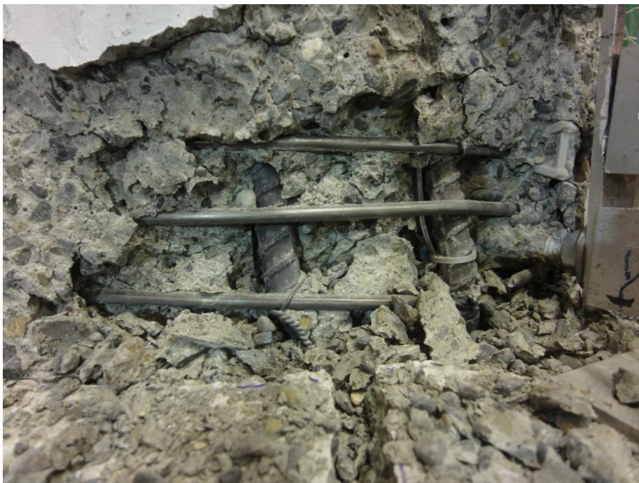
Figure C-0-18. DS-3 – First column spiral fractured at 6.88/-7.03 percent drift
