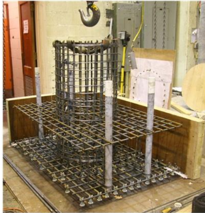
b). Shaft-Footing reinforcement
