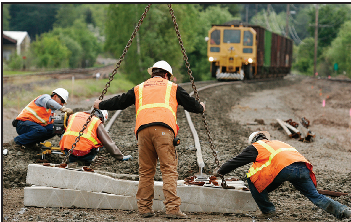
Working on the railroad
